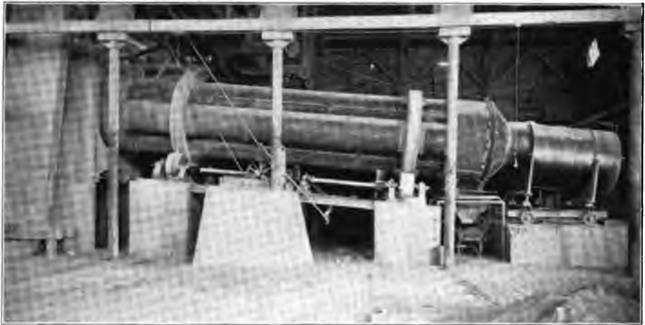
ARGALL ROASTING FURNACE, CYANIDE, COLO.
