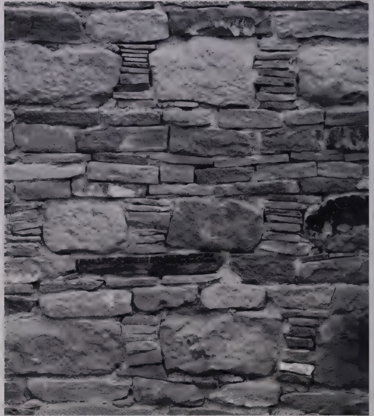
1127 An exquisitely constructed masonry wall at Pueblo Bonito, Chaco Canyon, that was then covered with plaster. A.D. 1011-1130.
