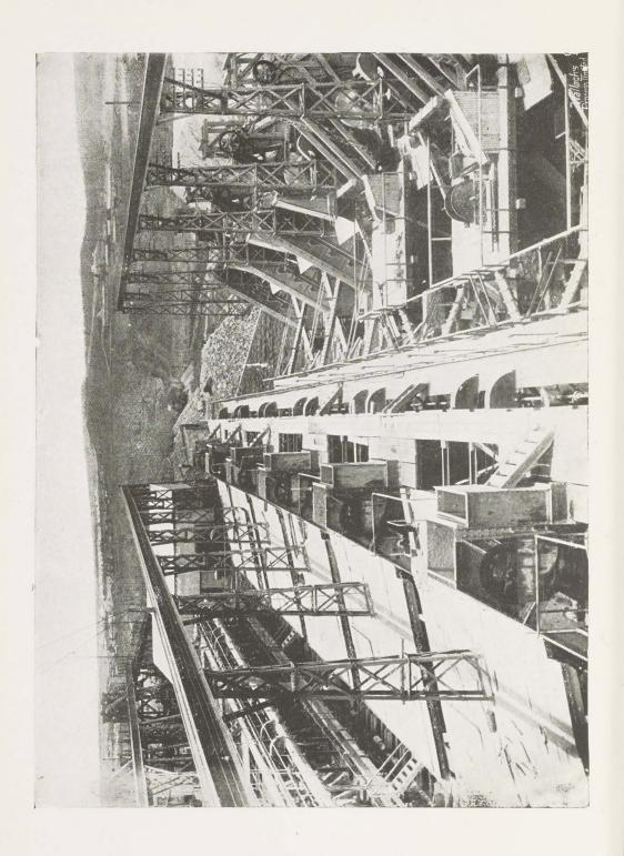
The discharge from the top pans passes through a set of 6 feet smooth rolls, which finally reduce the ground to 3/16", and thence into the bottom pans, the overflow from the bottom pans passing to the Tailings Elevators, which discharge the waste ground in the
