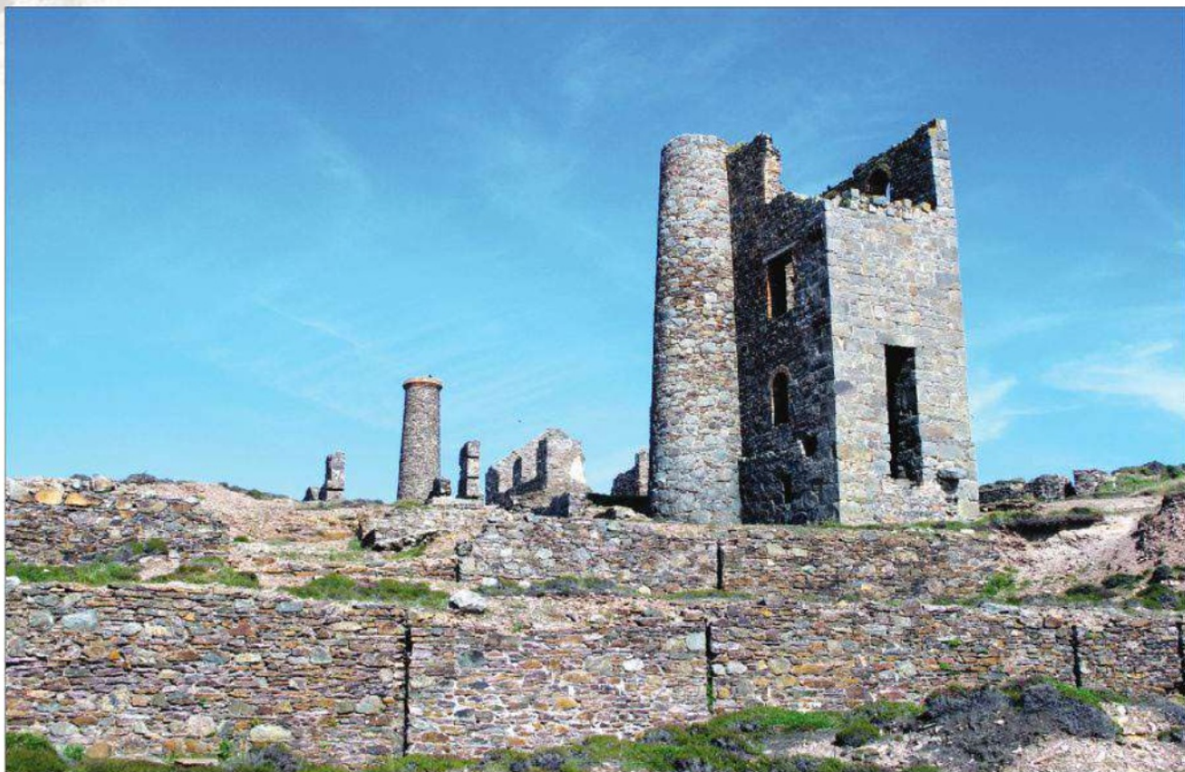
Cornwall's mines have long been abandoned, but an engine house and surface workings remain as stark reminders of a great mining past.
