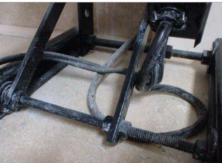
The 45° braces help prevent the vertical displacement of the boom support uprights.
