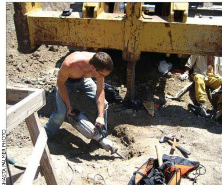
A jackhammer is a much more efficient tool for breaking up the overburden, but it requires a gasoline-powered generator to run.
