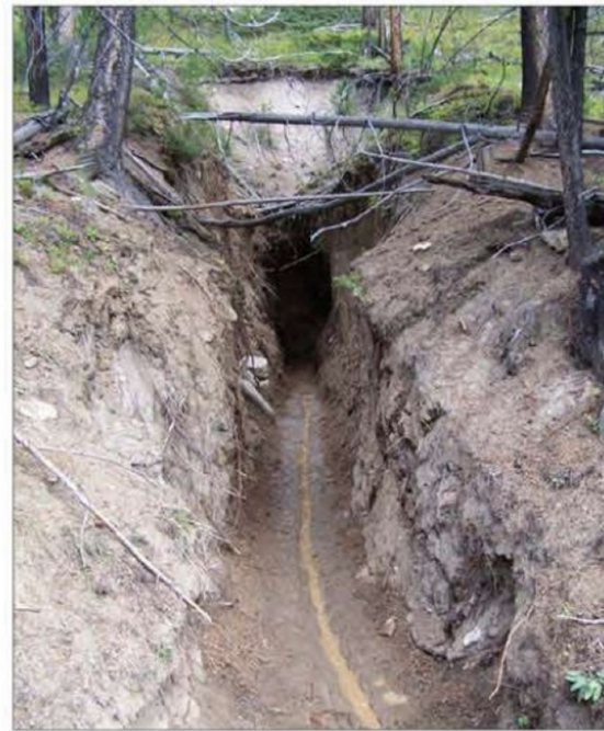
TOP: All the collapsed subsoil was removed back to hard rock to reopen this drift.
