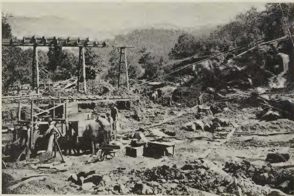
FIGURE 16. An old photograph (1897) of the ruby and rhodolite garnet diggings along Cowee Creek, North Carolina during the period when the mines were under the management of W. E. Hidden. Miners are digging gravel in the background which is then delivered to the washing rig at the left where crystals were separated from the worthless pebbles. The man in the foreground is seated at the sorting table. Courtesy U.S. Geological Survey.
