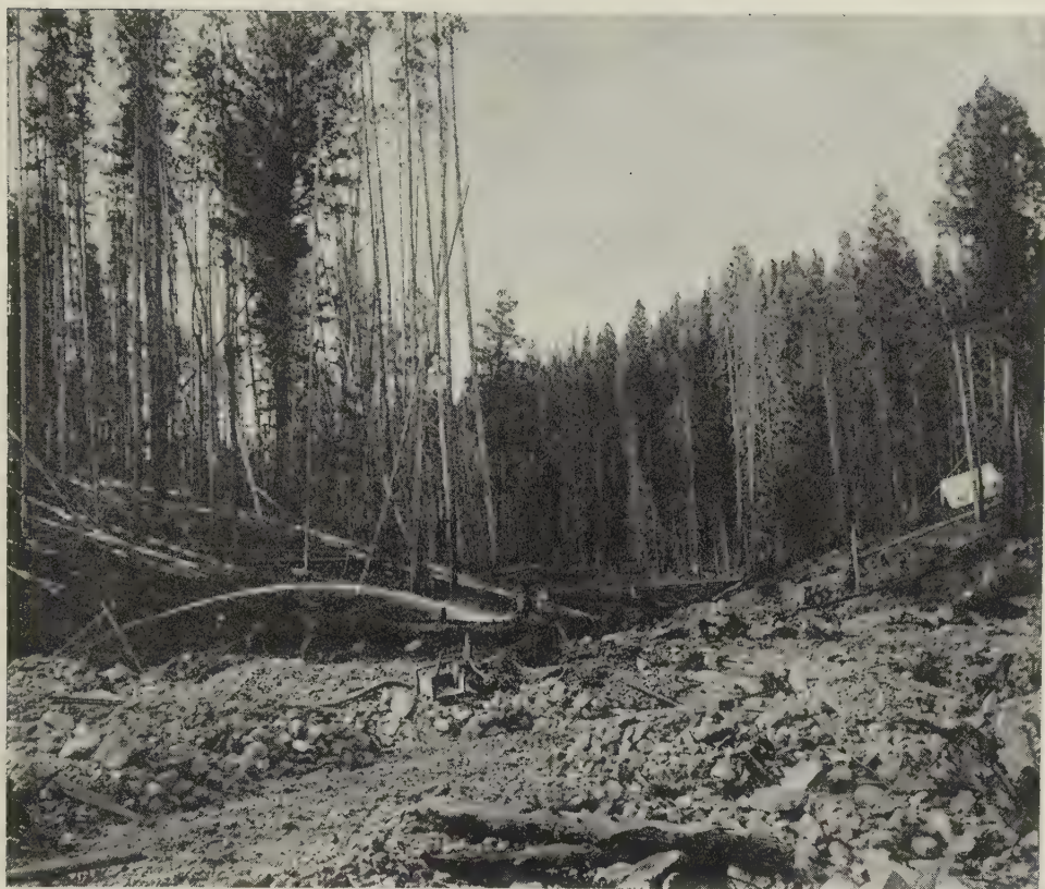
FIGURE 18. American Gem Syndicate sapphire mine on the west fork of Rock Creek, 20 miles southwest of Phillipsburg, Montana. Photo taken about 1914. The process of hydraulic mining for sapphire in the creek bed gravels is illustrated and involves the use of a head of water taken from the dam in the background and directed by a hose against the sapphire-bearing soil and gravel. Courtesy U.S. Geological Survey.
