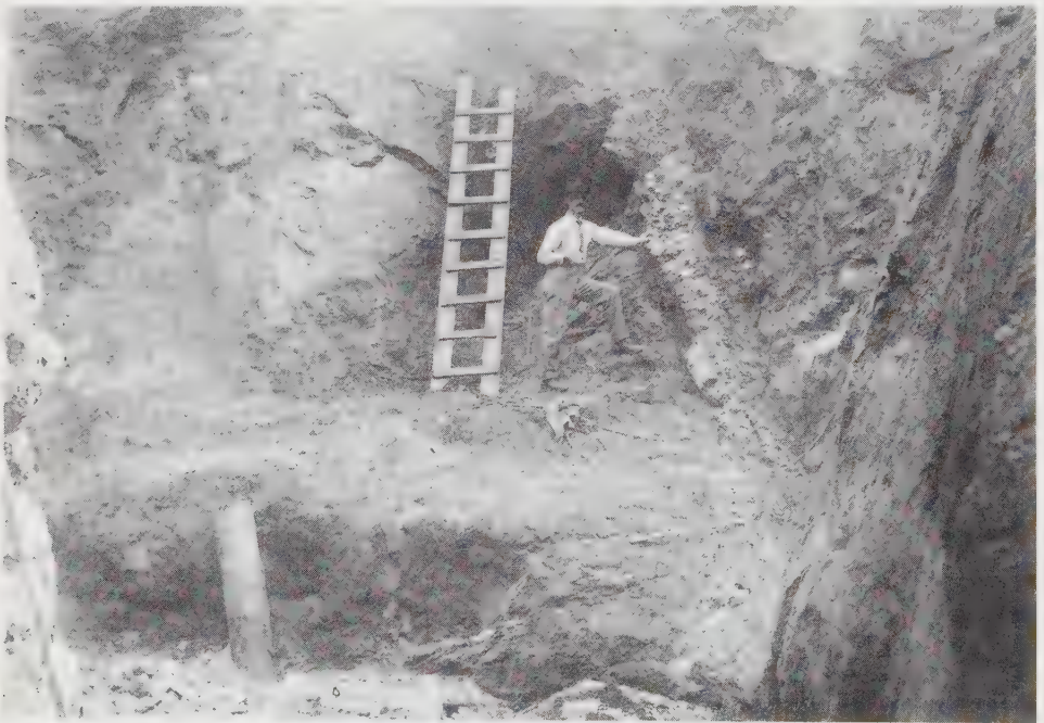
FIGURE 22. The Turner Emerald Mine near Shelby, North Carolina, September 27, 1912. The emerald-bearing pegmatite dike is to the right and appears as a whitish crumbly feldspar streak passing from the top of the excavation to the bottom past the sledge hammer. The decomposed nature of the country rock is apparent in this photograph. Courtesy U.S. Geological Survey.
