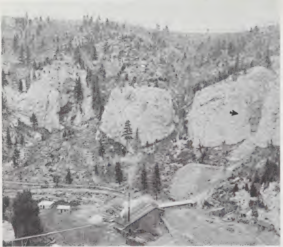
FIGURE 17. The American Sapphire Mine in Yogo Gulch, Montana in 1912; view looking northeast across the gulch. The steep cliffs are limestone and is the rock in which the sapphire-bearing dike is intruded. At the extreme right as marked by the arrow, the narrow defile created by removal of the dike rock is still to be seen. Courtesy U.S. Geological Survey.
