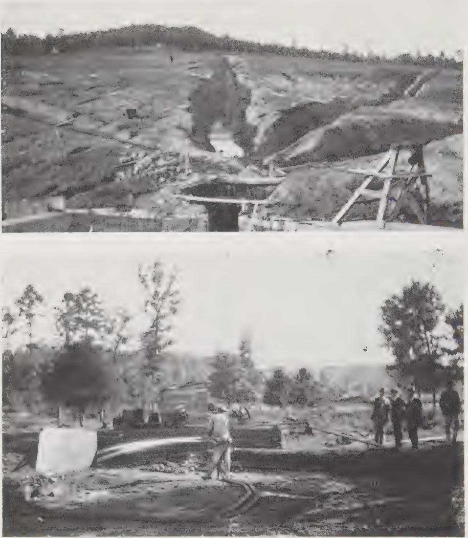
FIGURE 11. Two views of the diamond mine near Murfreesboro, Arkansas in October, 1923. The upper view shows a portion of the kimberlite outcrop cleared of vegetation and partially excavated by means of a dragline scraper. The bottom view shows one of the workmen washing some of the ground to separate the diamond crystals. Courtesy U.S. Geological Survey.
