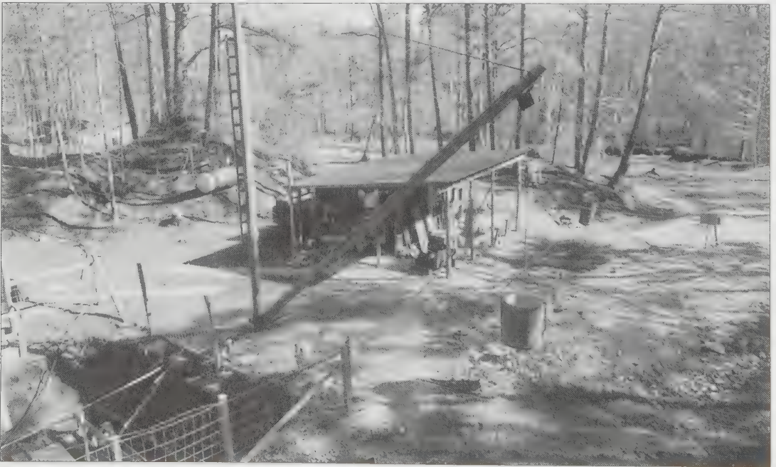
FIGURE 29. Morefield pegmatite mine near Amelia, Amelia County, Virginia, showing the old shaft and hoisting arrangements. Courtesy W. D. Baltzley, Powhatan Mining Co., Amelia, VA.
