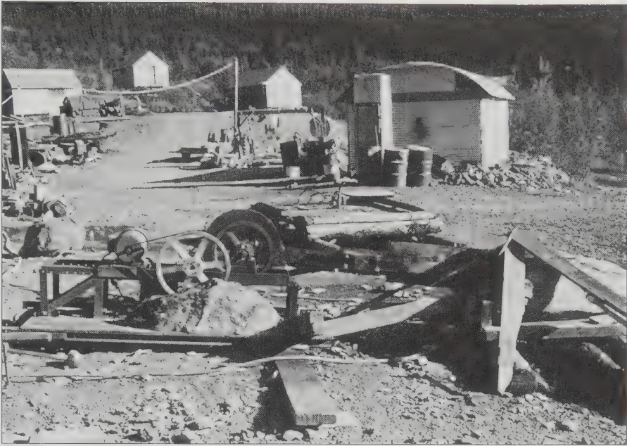
FIGURE 39. A 10-foot reciprocating saw used to section very large nephrite boulders of Dahl Creek, Alaska. Courtesy Oro R. Stewart.
