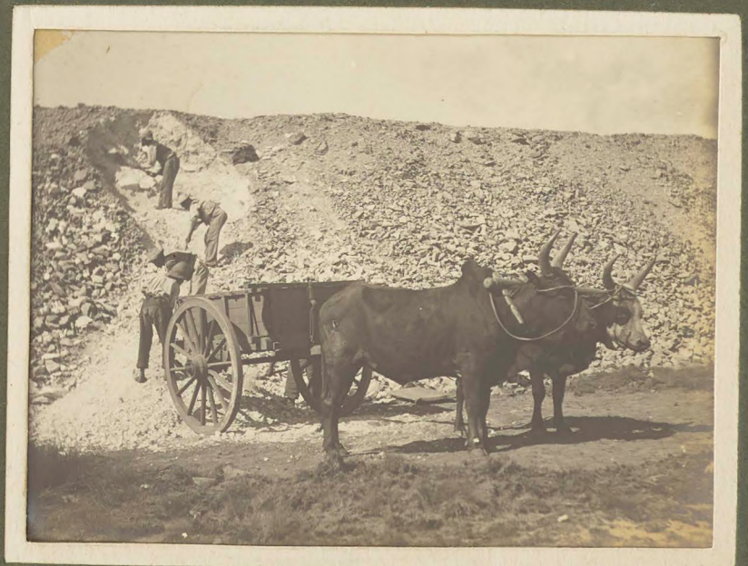
Removing Waste Rock, Windsor Mine Luspaards Vlei
