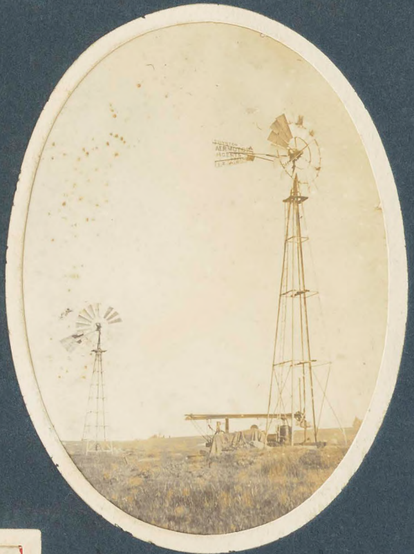
WIND MILLS for raising water for the Lepards del Mine
