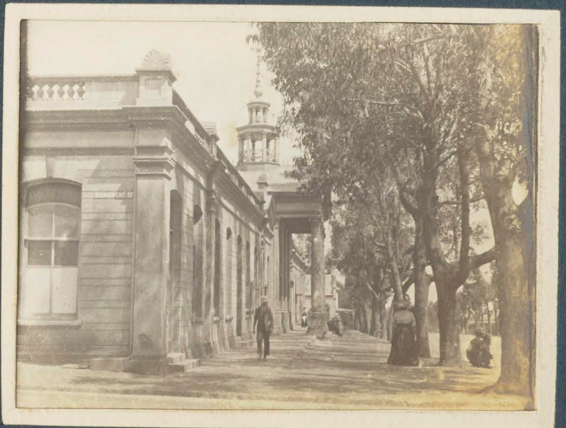
Court House Kragersdorp
