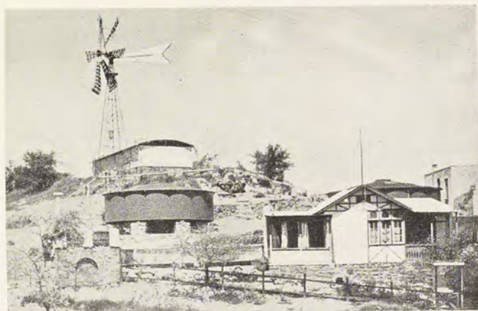
THE WATERWORKS, WINDHOEK.
