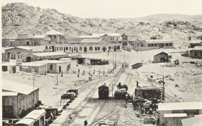
LUDERITZBUCHT RAILWAY STATION.
