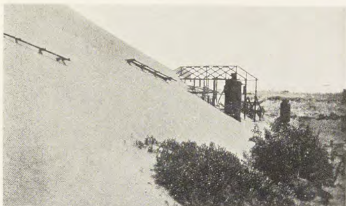
RUINS OF A JAM FACTORY AT SANDFISCHHAFEN, BURIED BY THE SHIFTING SANDS.
