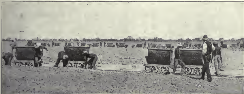
Loading Pulverized Blue Ground, De Beers Floors.
