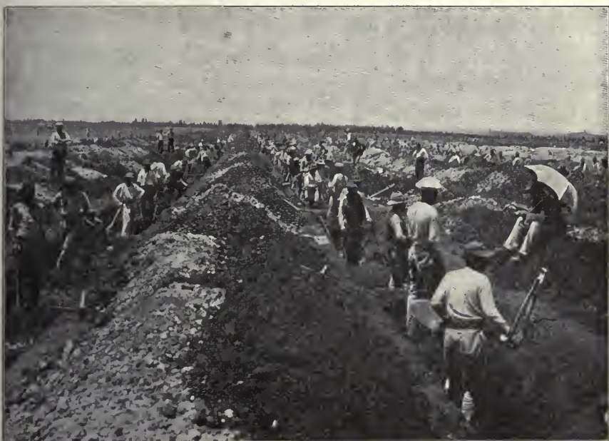
Preparing Trenches for planting Vines and Trees.
