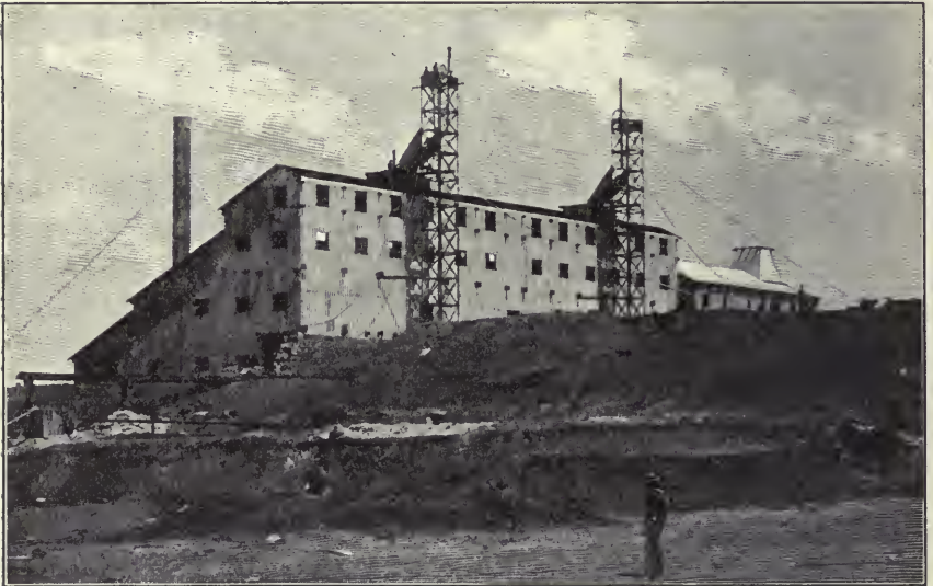
De Beers Crushing Mill, Back View.
