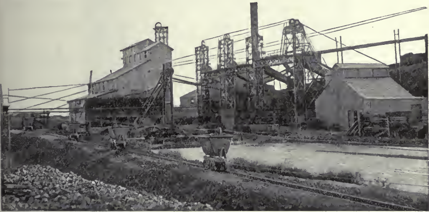
No. 2 Washing Plant, De Beers Floors.
