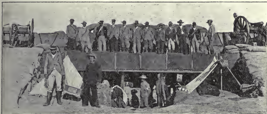
No. 2 Redoubt, near Kimberley Mine.
