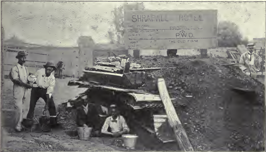
Shell-proof, constructed by the Public Works Department.
