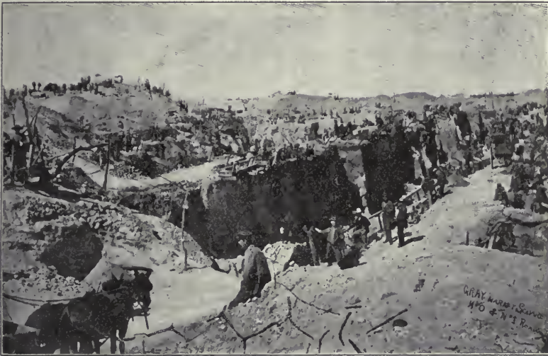
Kimberley Mine. (Showing workings in 1872. Subsidence cracks appear in the foreground.)
