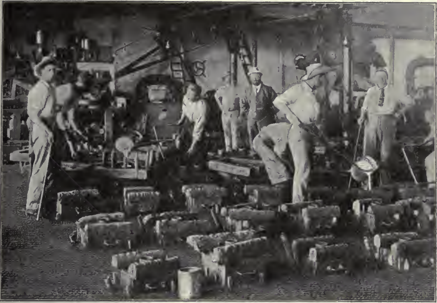
Casting Shells for Seven-pounders, De Beers Foundry.
