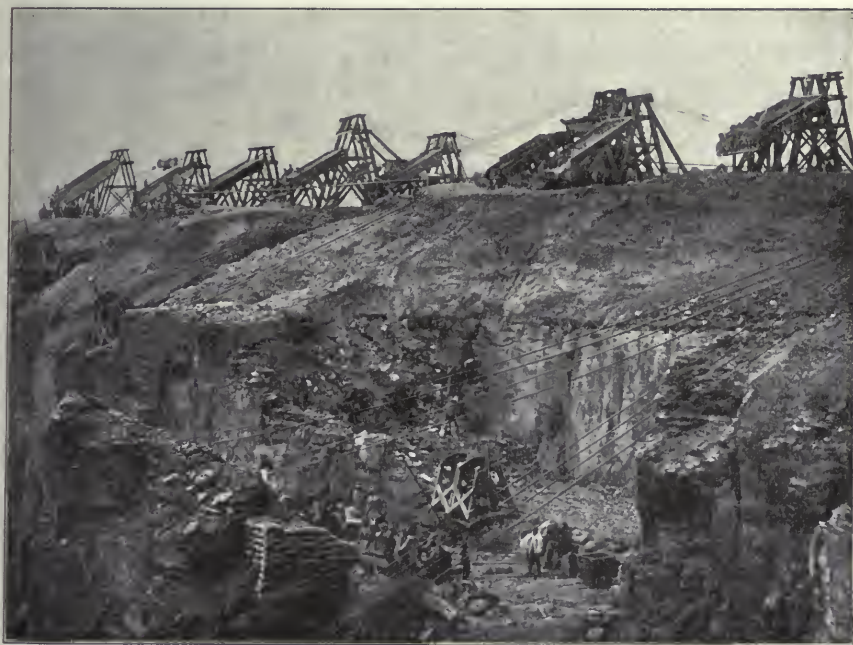
Aerial Trams and Surface Chutes, De Beers Mine, 1885.
