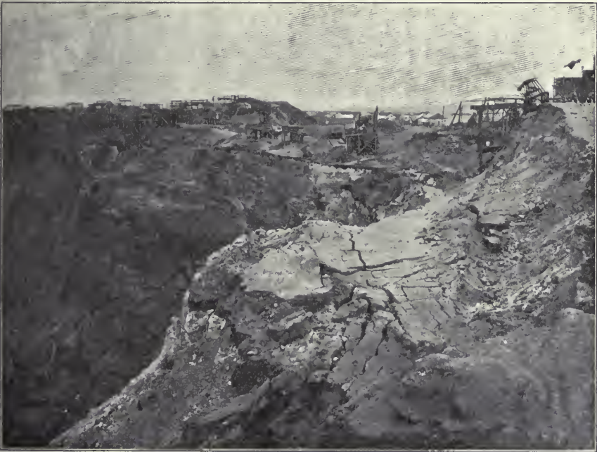
Kimberley Mine, showing how the Ground cracked before Subsidence.
