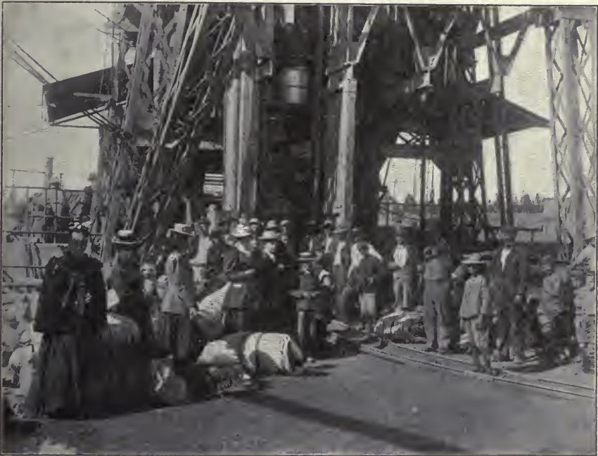
Double-decked Cage loaded with People and their Bedding being hoisted from the 1200-foot level of De Beers Mine.
