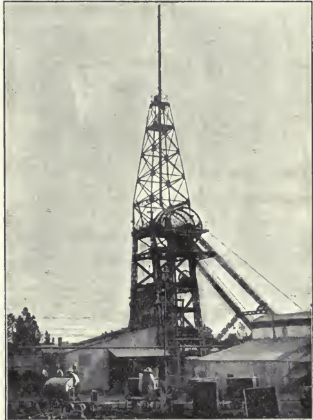
The Rock Shaft, De Beers Mine.
