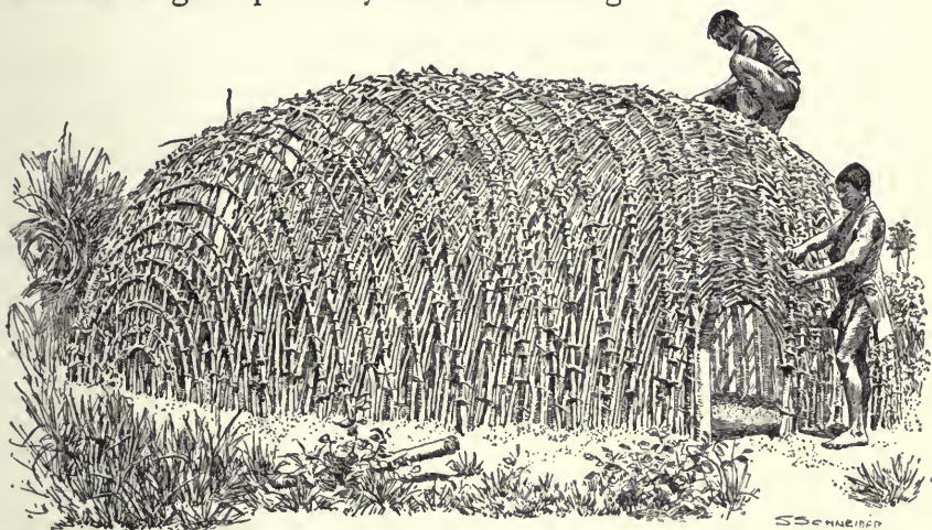
Zulu Hut in course of Construction.
