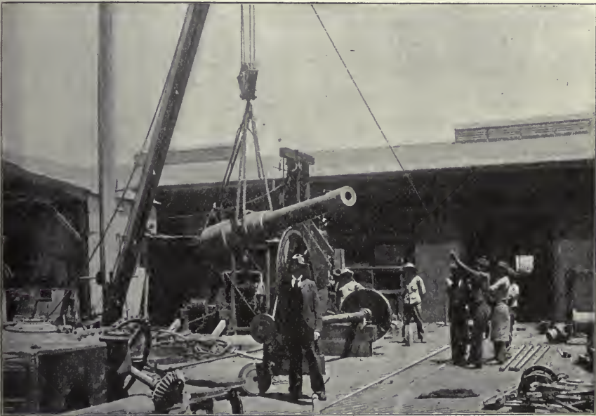
"Long Cecil" in course of Construction.
