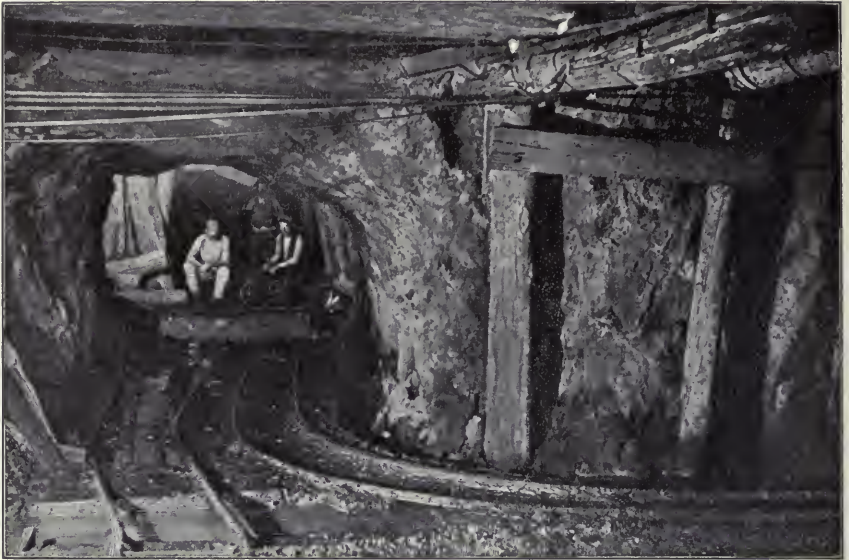
Timbered Tunnels at the 1000-foot Level, Kimberley Mine.
