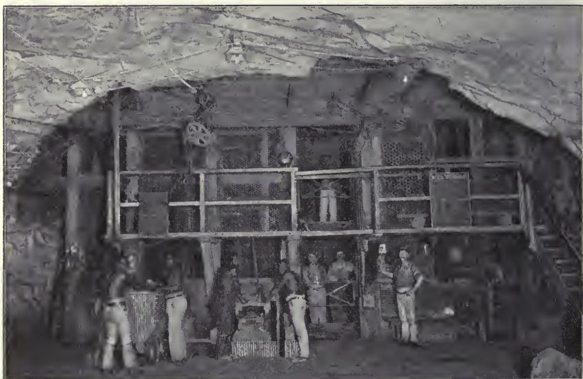
A Shaft Station.
