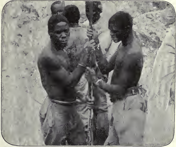
Natives drilling in the Open Mine.
