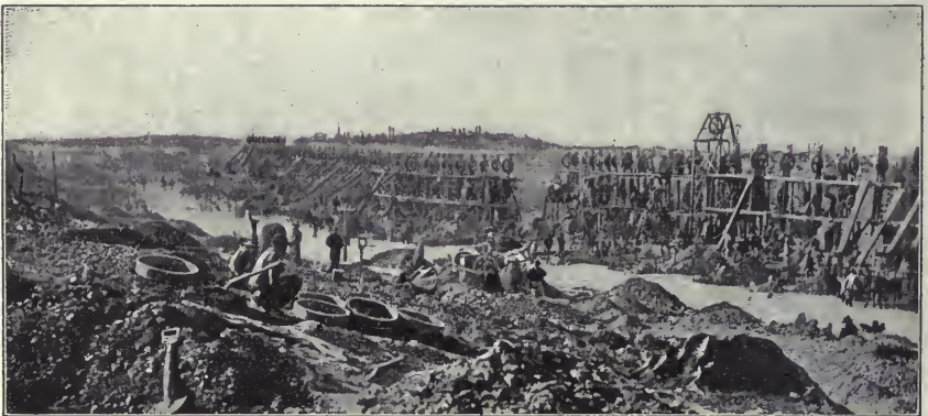
Back View of the Staging with Grooved Wheels, at Kimberley.
