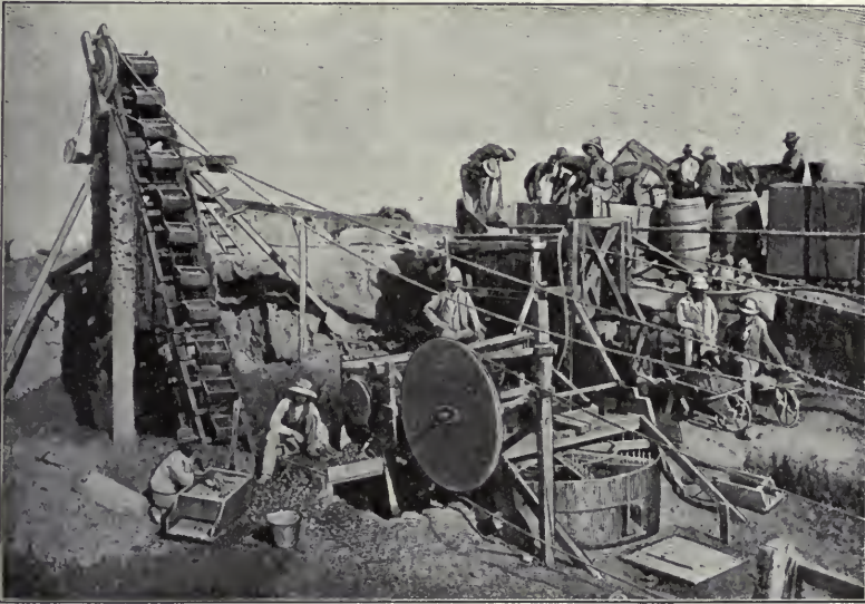
Steam Washing Gear, Kimberley Mine.
