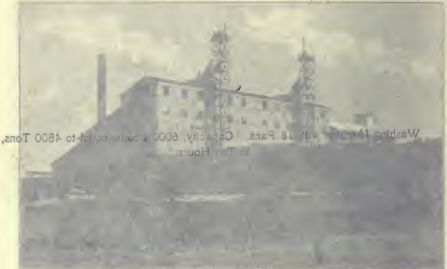
De Beers Crushing Mill, Back View.
