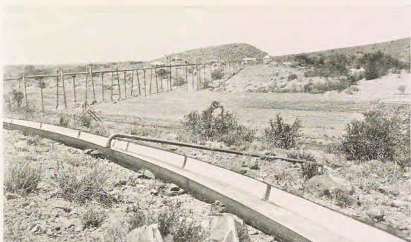
IRRIGATION : MAIN WATER FURROW AND LOCAL SYPHON
