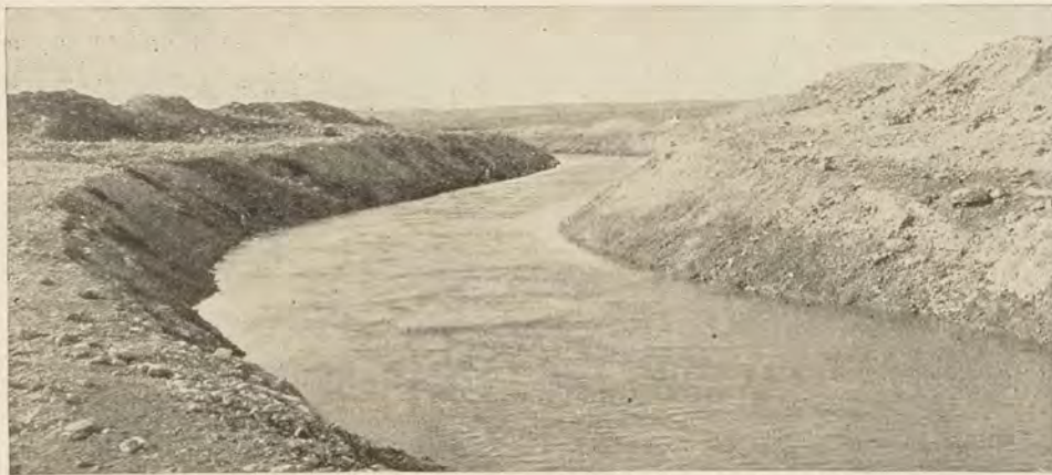
Irrigation Canal Showing Barrenness of Soil When Canal was Cut
