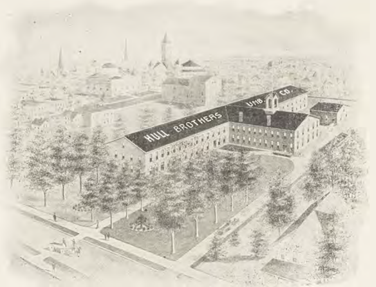
Factory at Norwalk, Ohio
