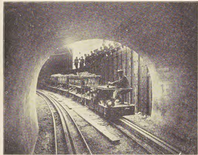
Coming to the surface with excavated material
