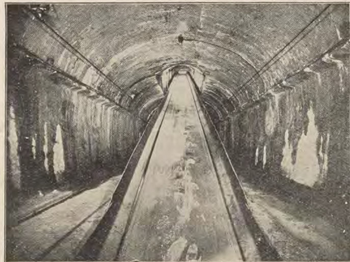
Belt conveyor to post office
