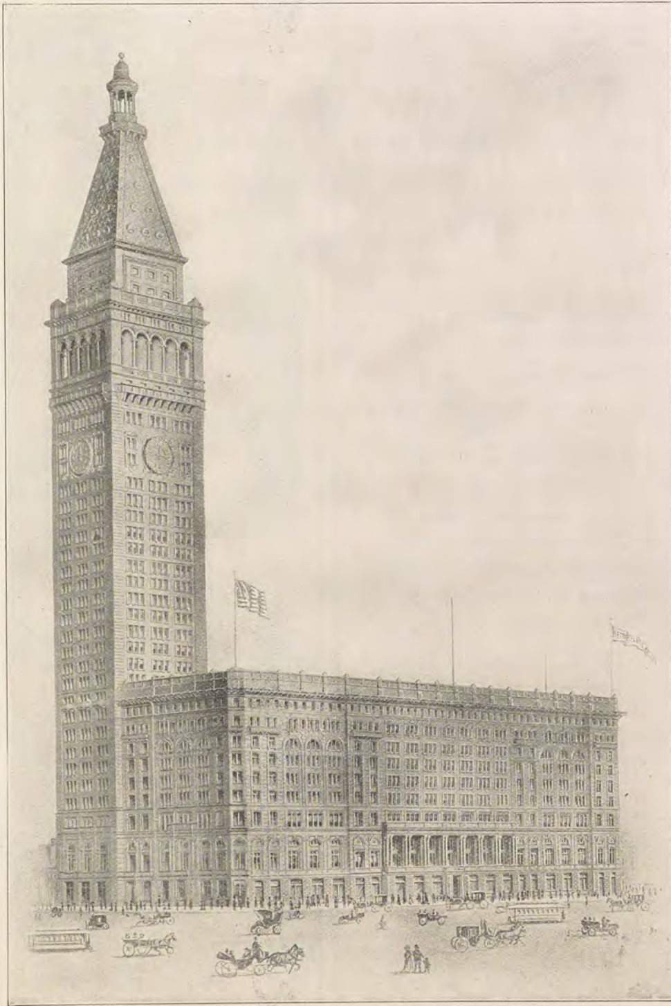
Metropolitan Life Insurance Building as it will appear when the new tower is erected. The tower will have 46 stories above pavement and two below. Extreme height from pavement, 658 feet.
