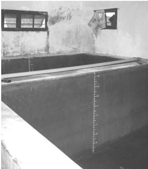
FIGURE 9.5 Large volume concrete tanks used for hatchery culture of Akoya pearl oysters, Li'an Bay, Hainan Province, China.
