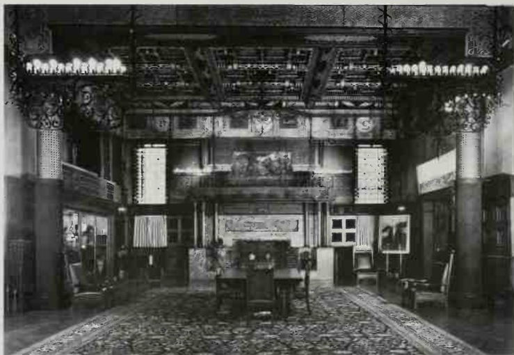
The Veterans Room in the Seventh Regimental Armory, New York City, designed by Tiffany, c. 1885. (Photo courtesy of The Historic Buildings Survey, National Parks Service; photographer Jack E. Boucher)
