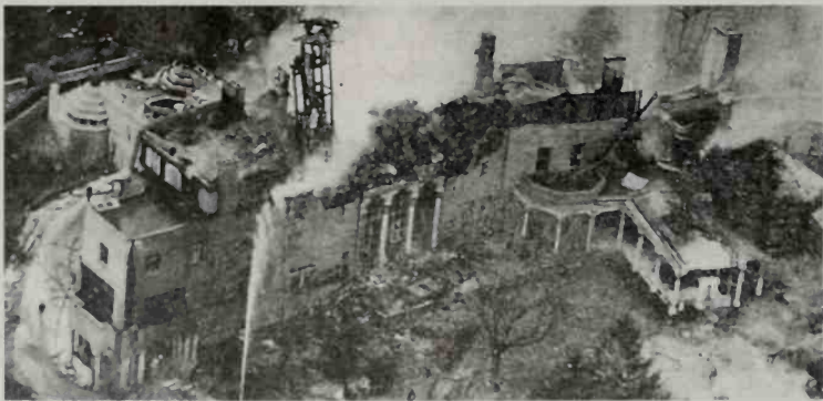
Fire at Laurelton Hall. 1957
