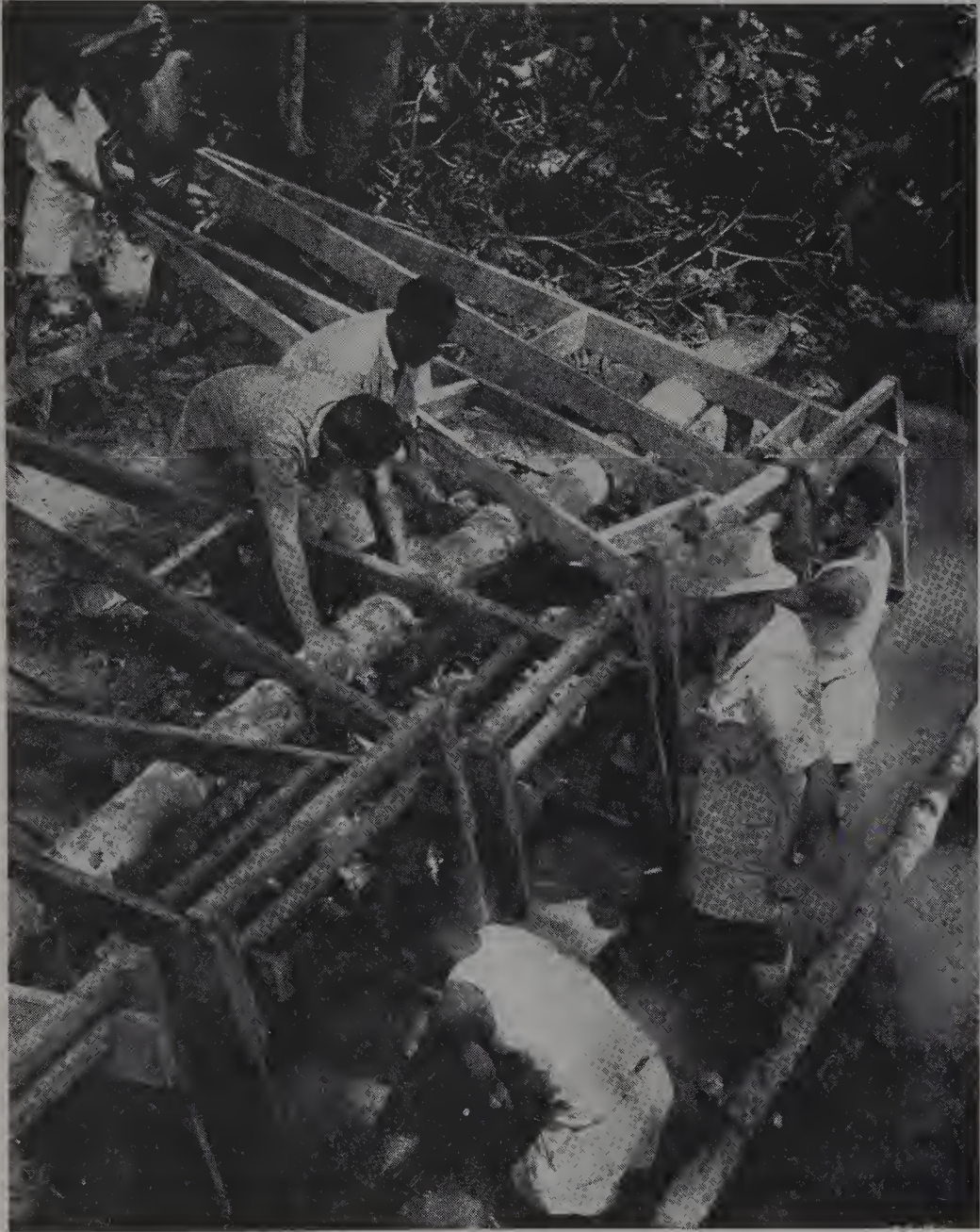
Figure 2.16. Diamondiferous gravel being washed in joplin jigs. The jigs are shaken by the long handles which causes the heavy density minerals to settle on the bottom of the jig screens
