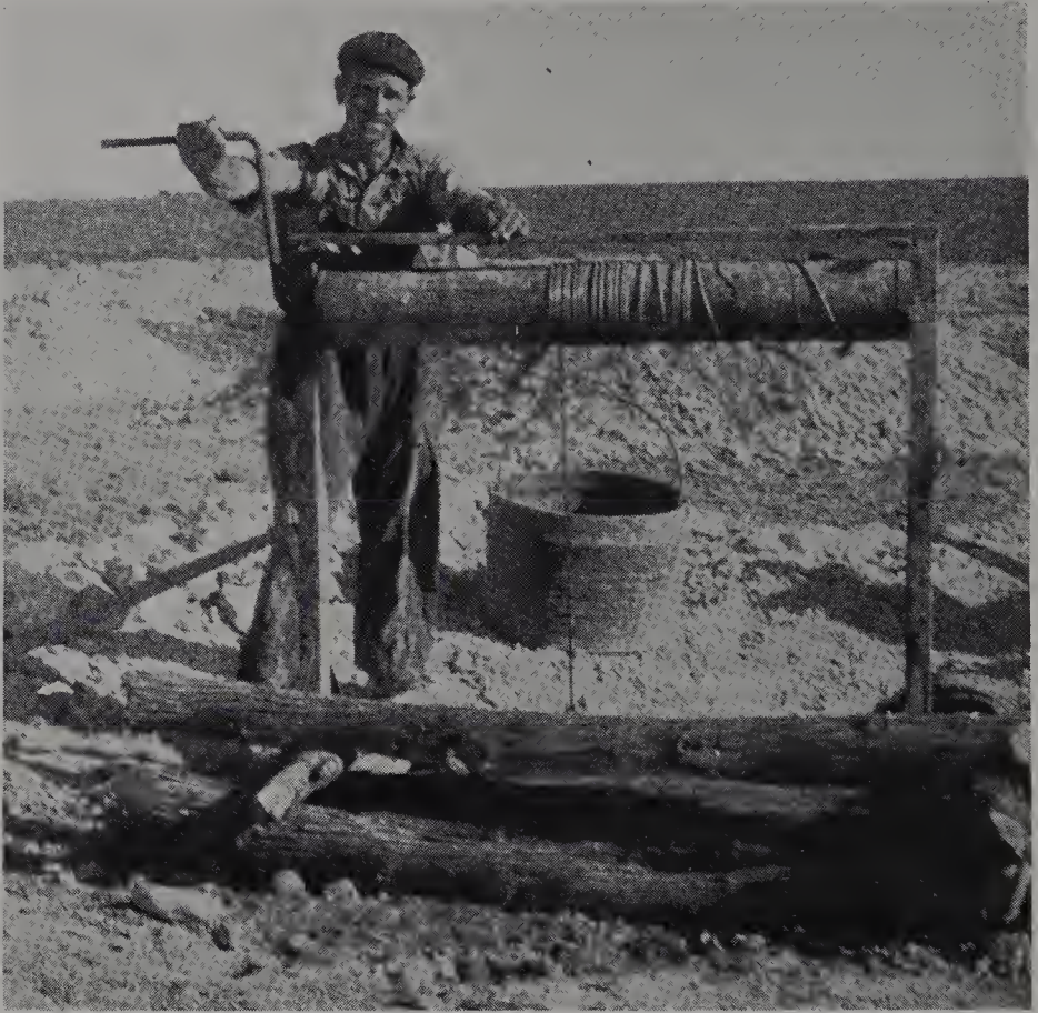
Figure 10.22. Opal mining at Andamooka. The miner turning the windlass is hauling up a bucket which a miner below ground has filled. In the background is an empty bucket
