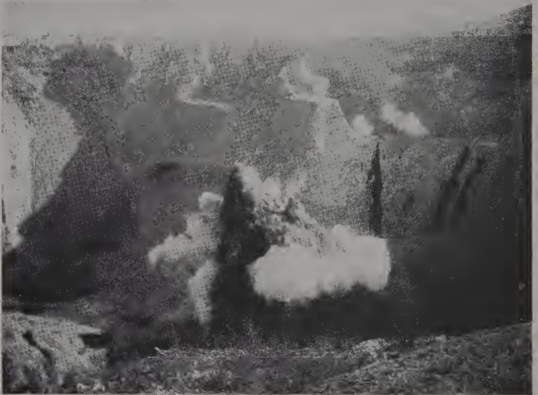
Figure 2.6. Blasting hard rock projecting into open mine at Bulfontein
