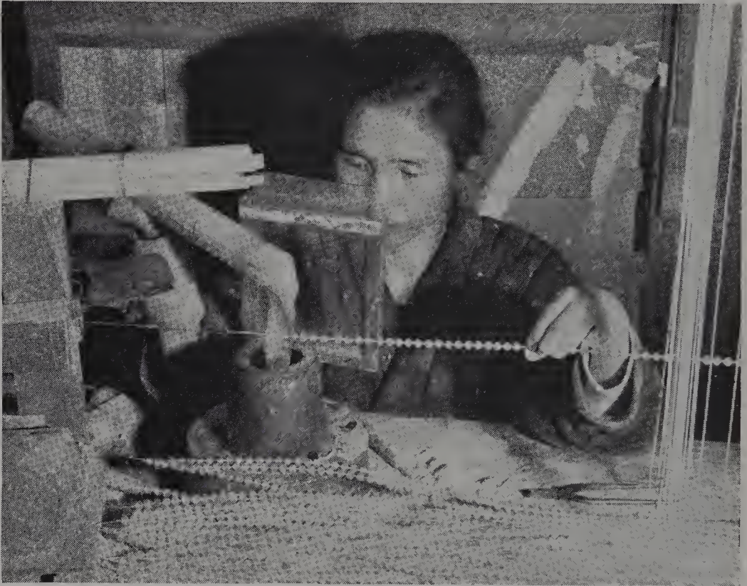
Figure 21.44. Forming the glass beads from easily fusible glass in Japan
