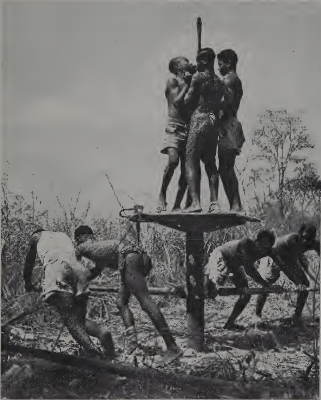
Figure 2.18. Manpower is used to operate the drill used in testing the depth of the overburden in the Central African Republic diamond fields
