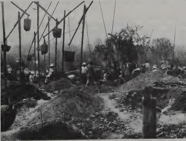
Figure 3.9 Washing the byon in the Burma ruby mines (by courtesy of J R H Chisholm, a former editor, Journal of Gemmology )
