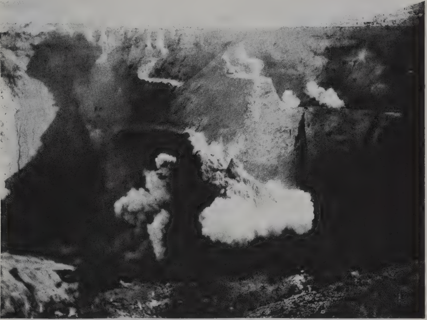
Figure 2.10 Blasting hard rock projecting into open mine at Bulfontein
