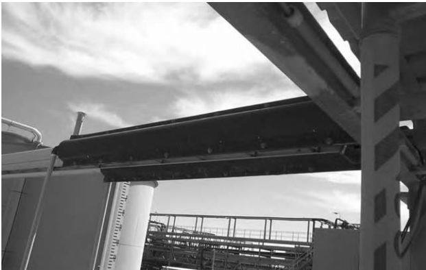
Fig. 8. Secondary containment for pipelines.
