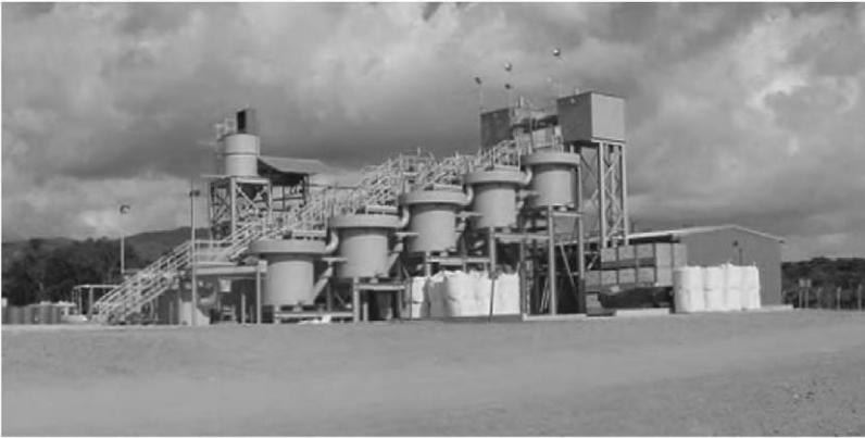
Fig. 5. Five-stage carbon adsorption column plant (CIC plant) built by Kappes, Cassidy & Associates for Glamis Gold's San Martin, Honduras project. There are two parallel column trains (one is behind the other in this view). The plant can process up to 900\text{ m}^3 of solution per hour, and is sized for an operation that processes up to 20,000 tonnes of ore per day.
