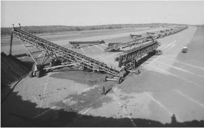
Fig. 3. Stacking system for capacity of 10,000 tonnes ore per day. Elements include stacker with extendable stinger; follower conveyor; cross conveyor; and several grass-hopper conveyors.
