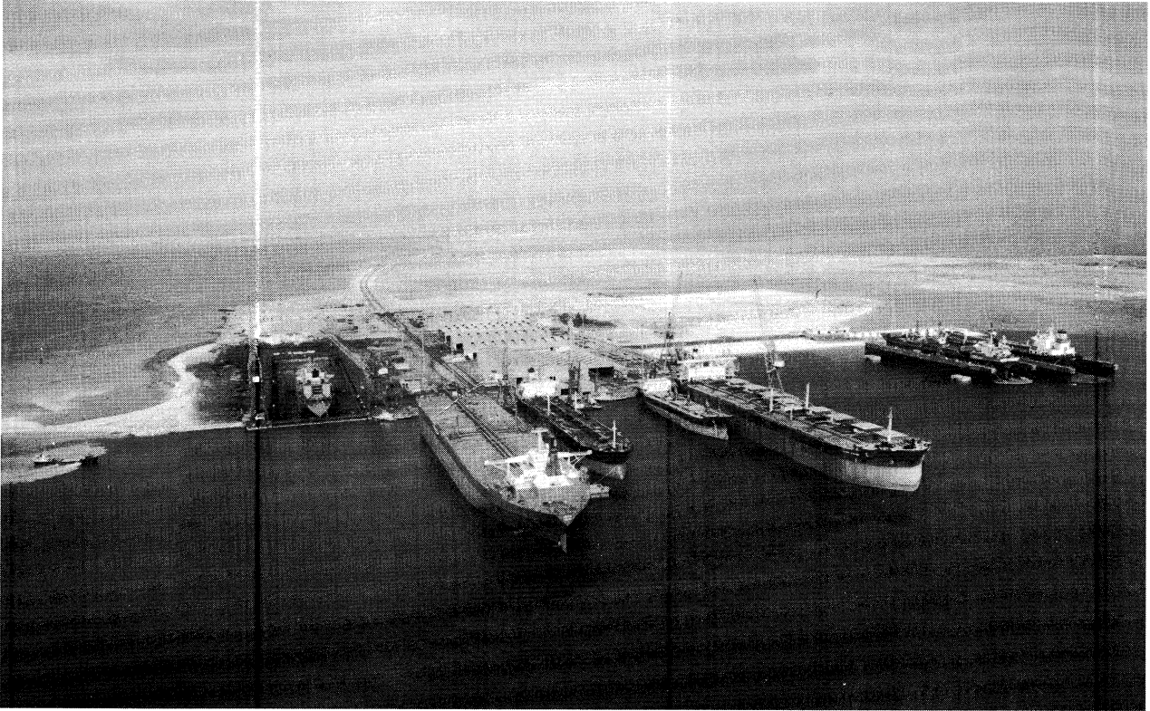
The Arab Shipbuilding & Repairyard Co. (ASRY) operations at Hidd, Bahrain. The drydock, in operation since 1977, can service ships up to 500,000 dwt. The two floating docks (far right) were purchased from Jacksonville Shipyards, a subsidiary of Fruehauf Trailer Corp. of the United States. The floating docks were placed in service in 1992 to accommodate ships up to 180,000 dwt.
