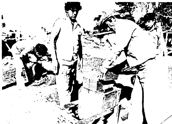
Removal of the ejected bricks.
