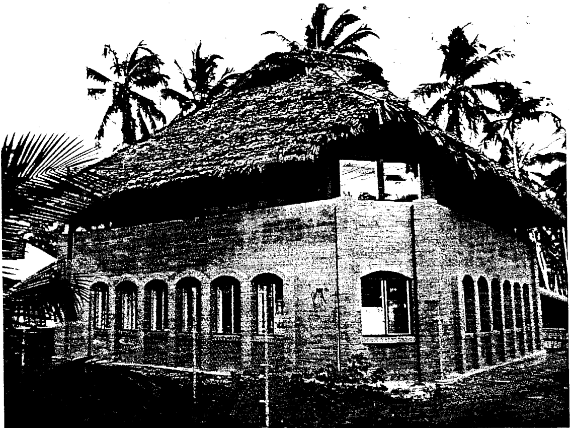
Town hall on the Isle of Mayotte, built with stabilized soil blocks, by CRATerre, Grenoble.
