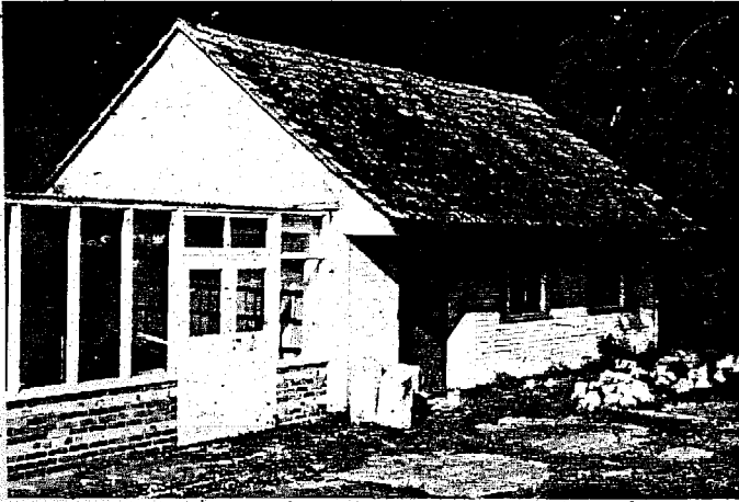
The experimental building which was constructed in 1950. The photograph was taken in October 1985.
