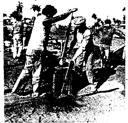
Position of lever just before compaction phase.
