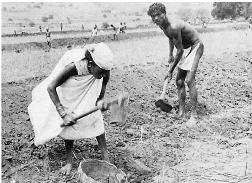
Figure 10-6 Farmers in central India building terraces with village-made hand hoes and head baskets. The state ministries of agriculture lay out and supervise the construction. (Courtesy Roy L. Donahue.)
