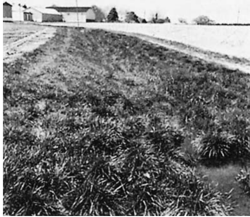
Figure 11–14 This V-shaped grassed waterway in North Carolina was vegetated with tall fescue in preparation for terracing the field. It provides a safe channel to carry runoff water from the terraces to a natural stream. (Courtesy USDA Natural Resources Conservation Service.)
