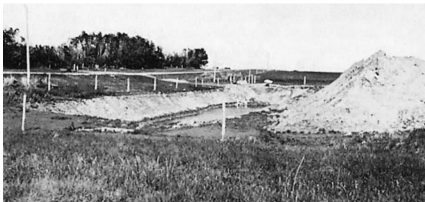
Figure 13-7 A dugout excavated in glacial till to impound water for livestock. A pump is located in the far corner. (Courtesy Canada-Manitoba Soil Survey.)
