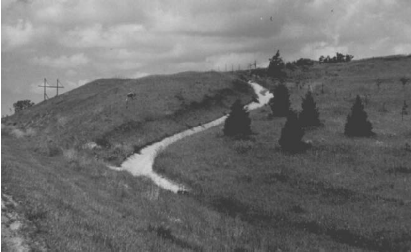
Figure 10–11 A concrete chute designed to carry runoff water safely down a slope to a road ditch at the bottom. (Courtesy F. R. Troeh.)
