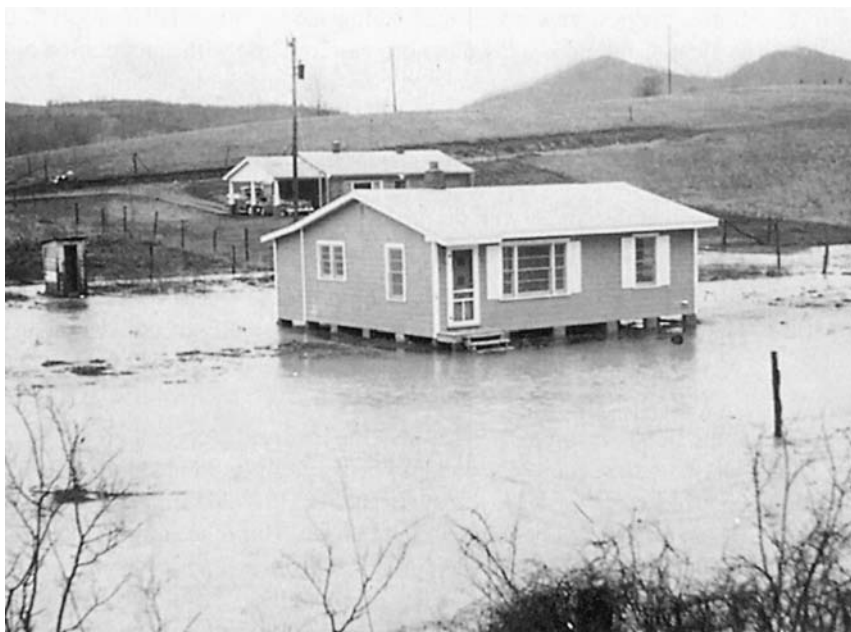
Figure 7-9 A zoning order based on soil maps would have prevented this house from being located on this area of Linside soil series. The soil is a Fluvaquentic Eutrochrept—the prefix “Fluv-” indicates the flooding hazard. (Courtesy H. C. Porter, Virginia Agricultural Experiment Station, Virginia Polytechnic Institute and State University.)
