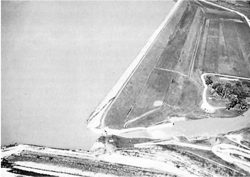
Figure 13–8 Lovewell Dam and Reservoir in north-central Kansas was built by the Bureau of Reclamation as an irrigation storage reservoir. The irrigation water discharge outlet and canal are in the foreground beside the spillway. Water was being discharged from the spillway when the picture was taken. (Courtesy USDA Natural Resources Conservation Service.)
