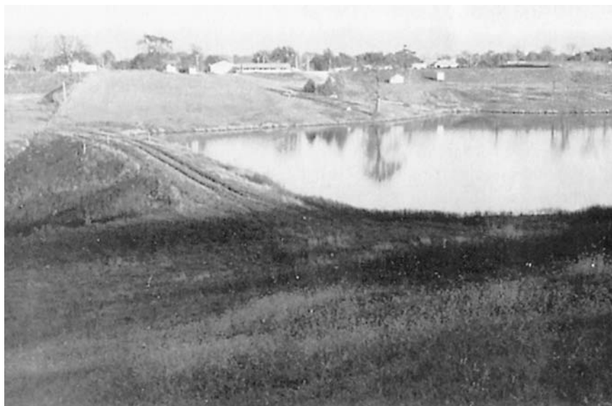
Figure 10-12 A Class B dam constructed in a gully to stop erosion and to provide a waterfront for recreation. (Courtesy USDA Natural Resources Conservation Service.)
