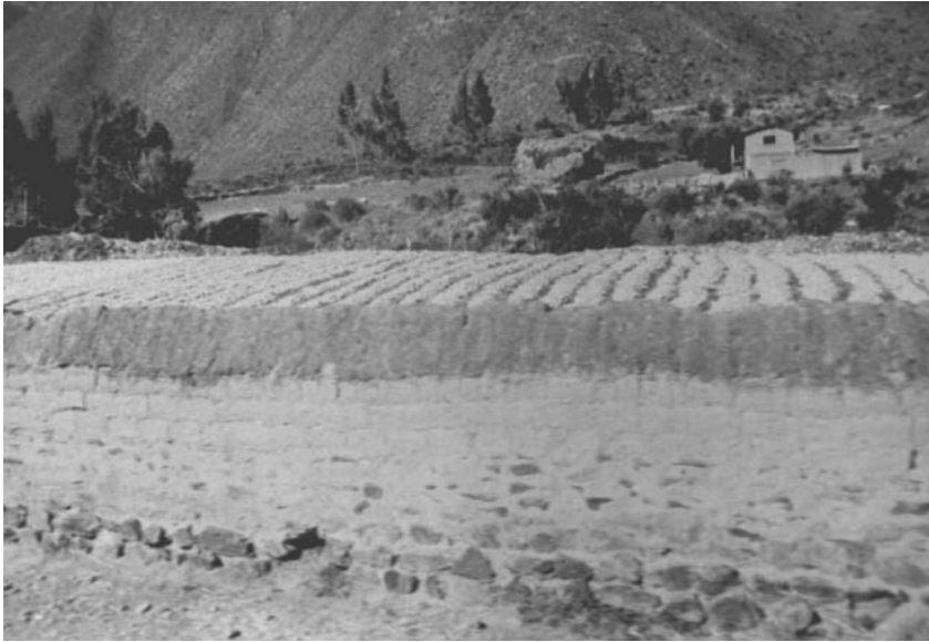
Figure 10-15 Rock wall revetment protecting a cultivated field from floods of the Urubamba River near Machu Picchu, Peru. (Courtesy F. R. Troeh.)
