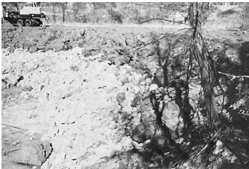
Figure 10-14 A toe protector to stabilize a streambank. The rock covers the bank from the low water level to the height of normal flood stage. (Courtesy Kansas City District, Corps of Engineers, U.S. Army, Kansas City, Missouri.)
