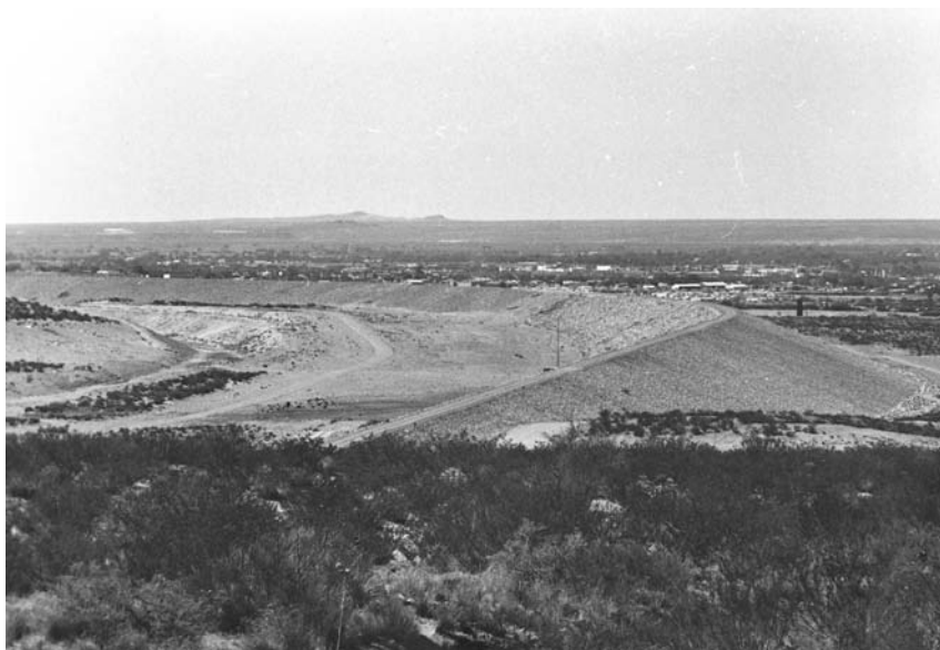
Figure 10-13 Flood control dam protecting Las Cruces, New Mexico. This is one of several similar structures built to impound runoff water from heavy rainstorms in the hills above the city. This structure is about 0.5-mi (1-km) long and has a road along the top. (Courtesy F. R. Troeh.)
