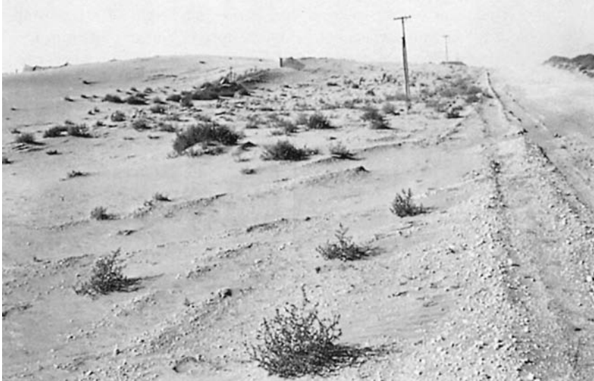
Figure 5-4 Wind erosion sediments have buried three snow fences erected to protect the road at the right of this picture. The surface of the dunes over the snow fences is 3 to 10 ft (1 to 3 m) above the former ground level. (Courtesy USDA Natural Resources Conservation Service.)
