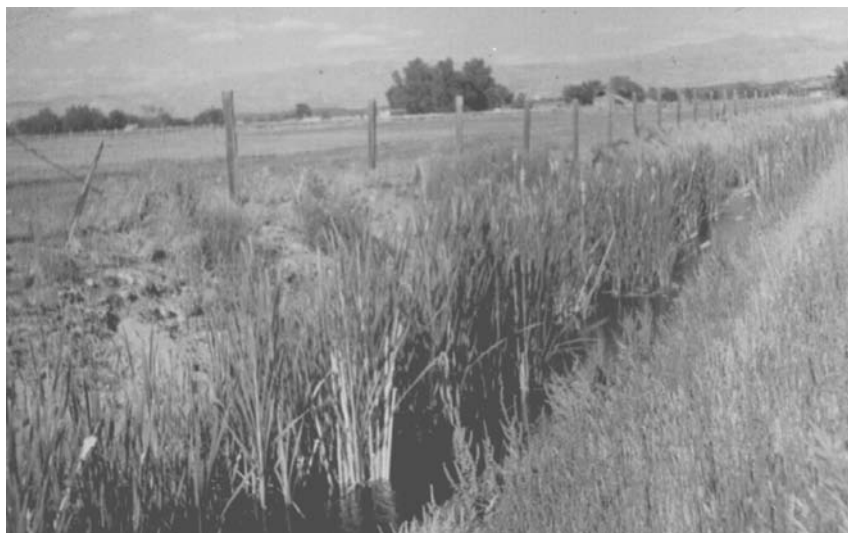
Figure 14-10 Vegetation stabilizes the banks of this drainage ditch, but the vegetation growing in the water slows the flow and raises the water level. (Courtesy F. R. Troeh.)
