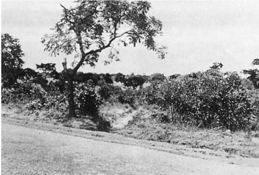
Figure 10–8 A diversion ditch in Nigeria designed to carry water from a highway ditch safely away from the right-of-way. Spreading the water on naturally vegetated sites dissipates its energy. (Courtesy J. A. Hobbs.)
