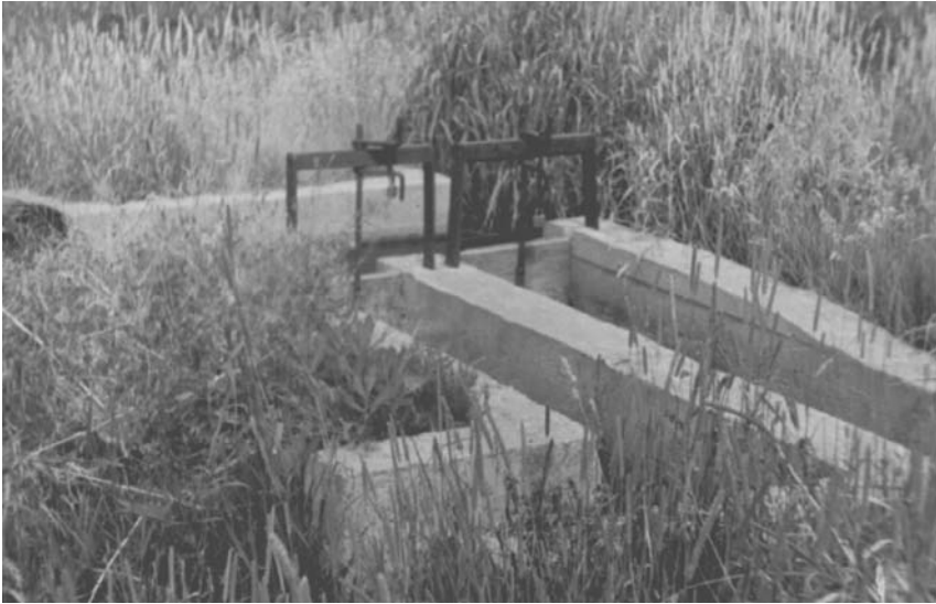
Figure 15–8 A division box for diverting water in any of three directions. (Courtesy F. R. Troeh.)
