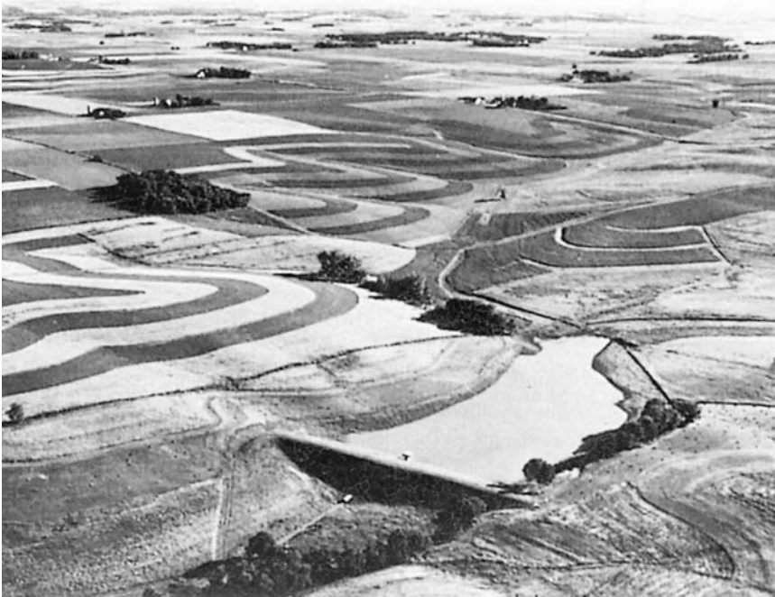
Figure 11-18 This large pond is part of the West Willow Creek Watershed project in Minnesota. It is designed to store 200 ac-ft (250,000 m 3 ) of water from a 2000-ac (800-ha) drainage area. Its banks are stabilized with adapted vegetation. (Courtesy USDA Natural Resources Conservation Service.)
