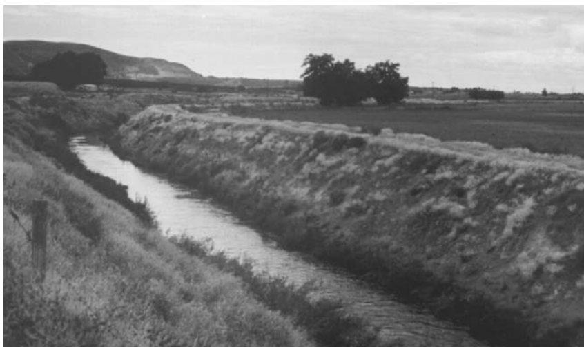
Figure 14-9 This 20-ft (6-m) deep ditch in Idaho serves as an overflow for irrigation water if the canal above gets too full, as an interceptor for seepage water, and as an outlet for drainage systems in the valley. (Courtesy F. R. Troeh.)
