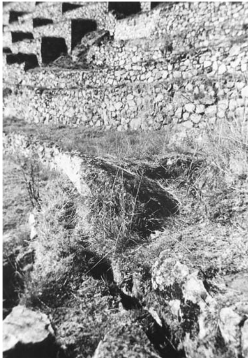
Figure 2-8 Rock-faced bench terraces constructed by the Incas at Machu Picchu, Peru (the “Lost City of the Incas”). The dark channel in the foreground carried irrigation water to the terrace. (Courtesy F. R. Troeh.)
