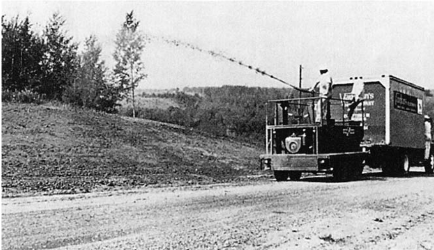
Figure 11-2 Seeding a roadcut by blowing a slurry onto the area. (Courtesy USDA Natural Resources Conservation Service.)
