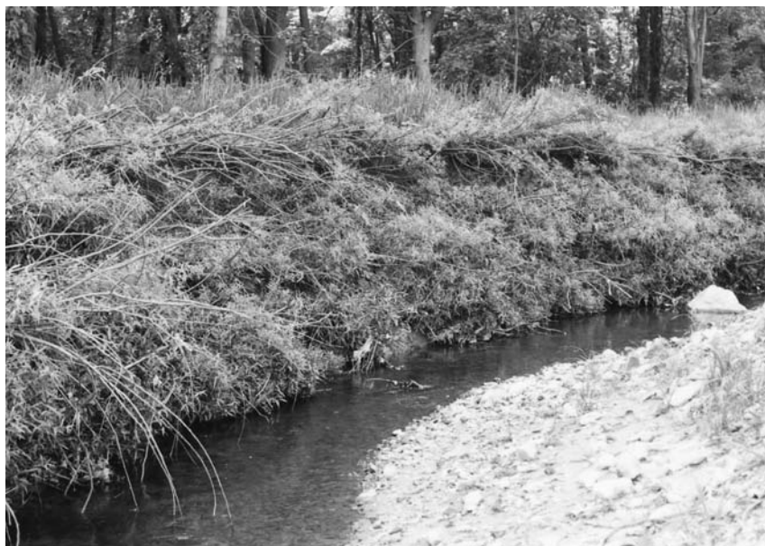
Figure 11-16 This streambank in Virginia was stabilized by planting woody cuttings. The shrubs next to the water are forsythia; the trees are willow and cottonwood. (Courtesy Northern Virginia Soil and Water Conservation District.)
