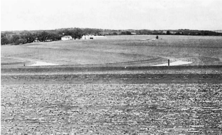
Figure 10-9 A terrace system in Kansas with tile inlets. Water drains through the black riser pipes in the terrace channels. This area received 9 in. (230 mm) of rain in 3 hours the day before the photo was taken. (Courtesy USDA Natural Resources Conservation Service.)
