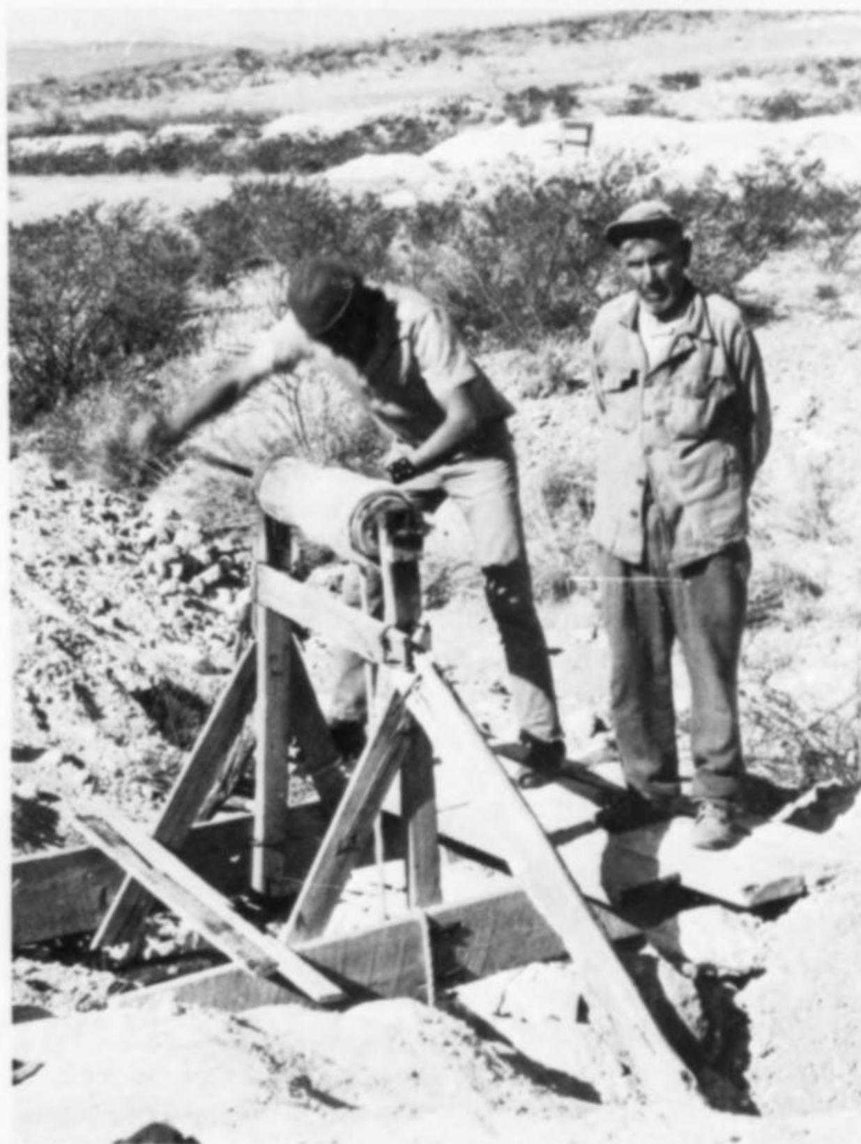
Figure 7. Geode mining downdip where it is necessary to dig through up to 10 m of overburden before striking the "productive zone." A man is lowered into the hole in a bucket that is then used to haul out debris and geodes.
