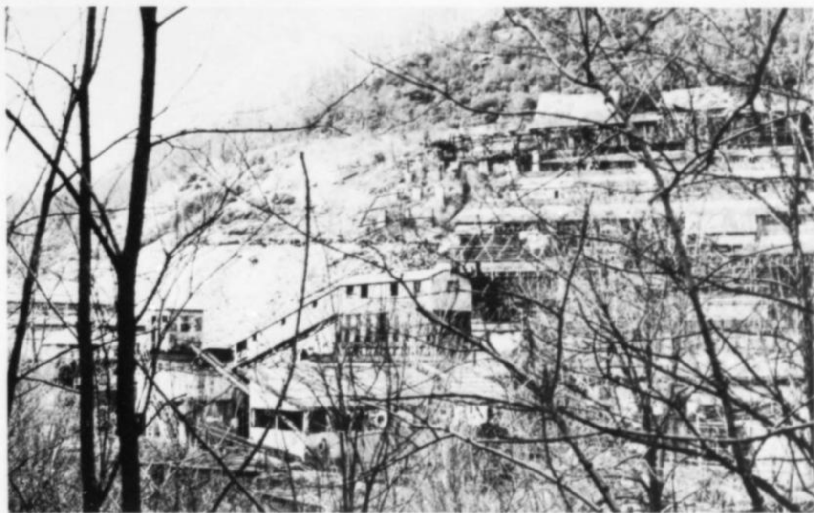
Figure 5. The Boccheggiano mine, abandoned installations, in 1977. Photo by P. B. Scortecci.
