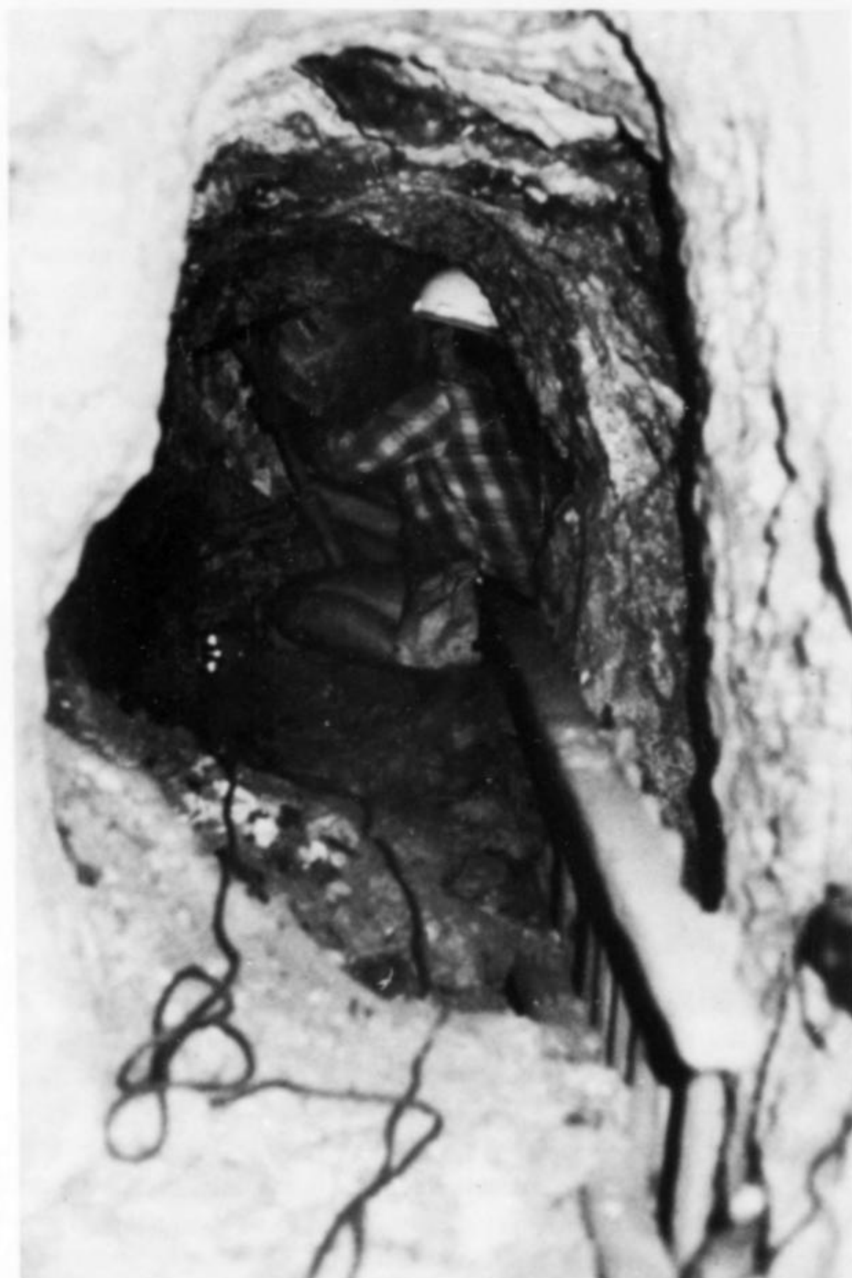
Figure 8. Working at the face of No. 2 adit, Sir Dominick mine. The large stope connecting levels two and three is immediately to the right of the ladder.
