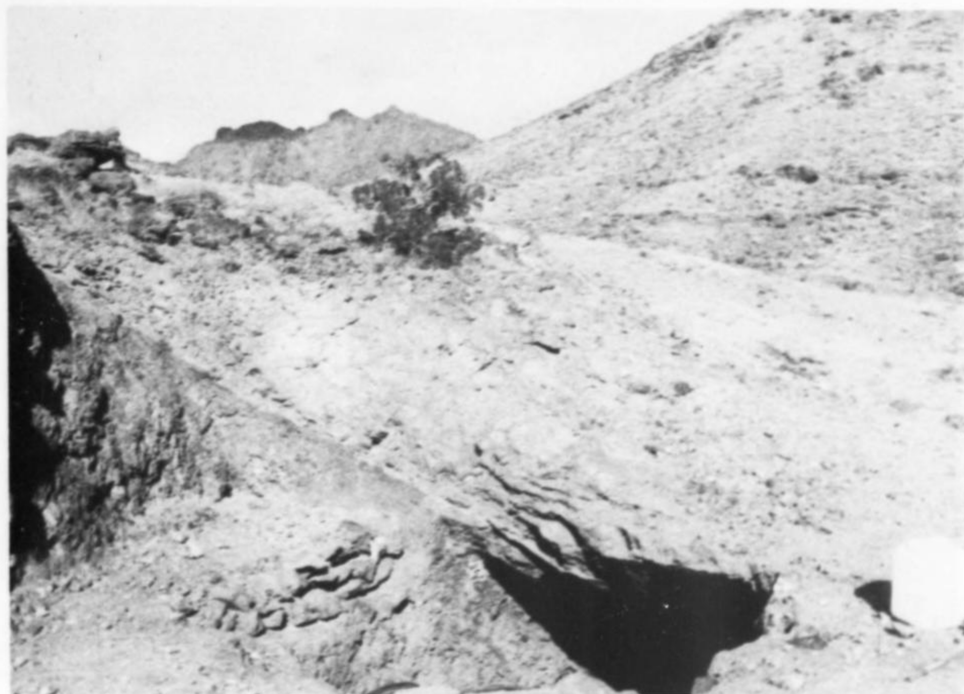
Figure 3. Entrance to the Hamburg mine. Note the fault contact which forms the hanging wall of the mine. The Princess mine is just over the first rise. Photo by the author.
