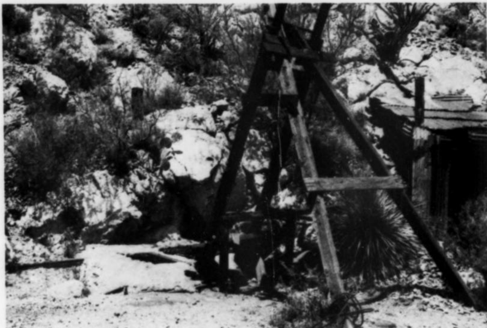
Figure 5. Entrance to the Defiance mine, a steep 60° incline topped by a concrete cap and small headframe. Photo by the author.
