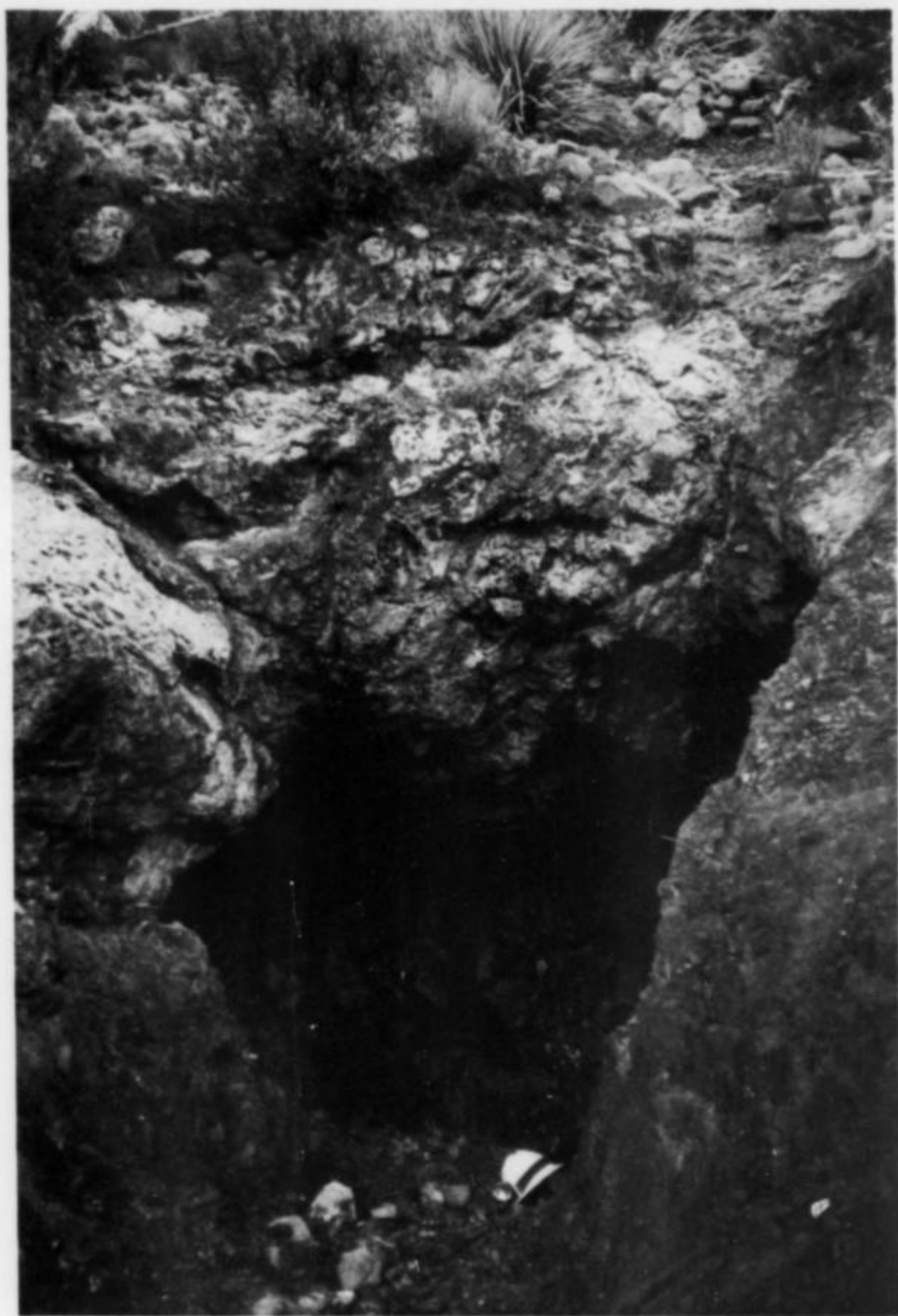
Figure 4. The entrance to the upper adit, showing diabase (right) in contact with brecciated limestone (center).
