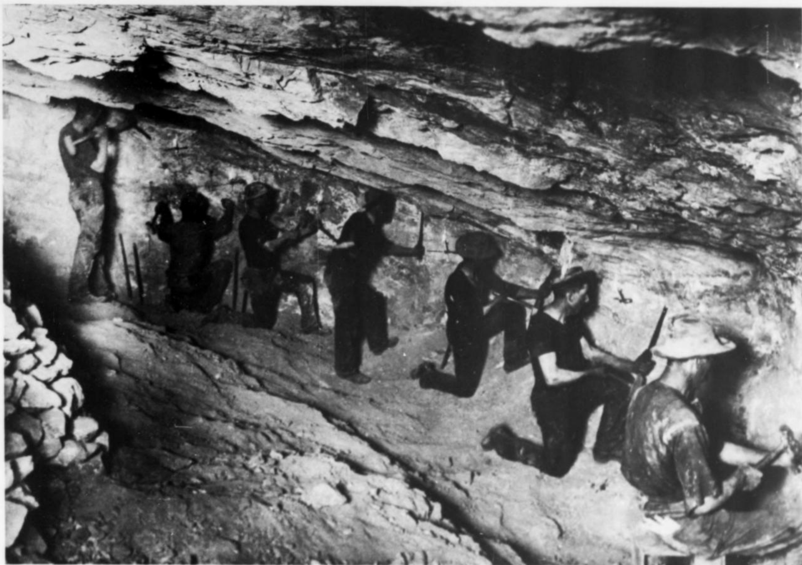
Figure 5. Miners single-jacking in a 5-foot thick vein of argentiferous galena on the 500-foot level of one of the Tombstone Consolidated Mines Company's mines in 1904. Photo courtesy of the Arizona Historical Society.
