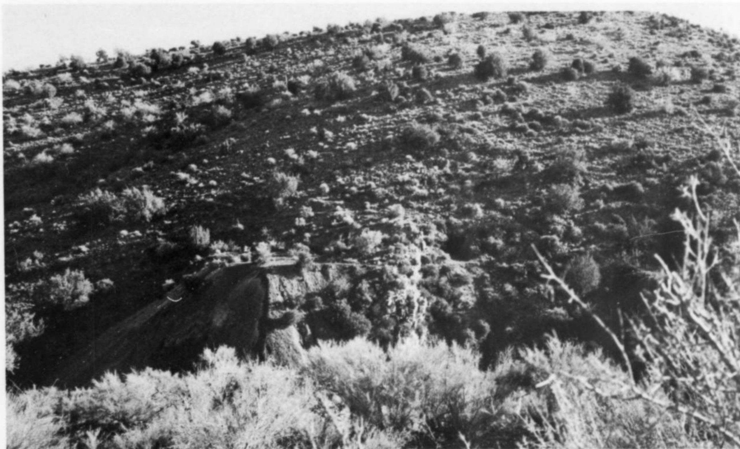
Figure 3. A view looking south toward the C. & B. mine dump, showing the open stope just behind the dump. The entrance to the upper workings is just to the right of the dump, and a short caved adit is farther to the right.
