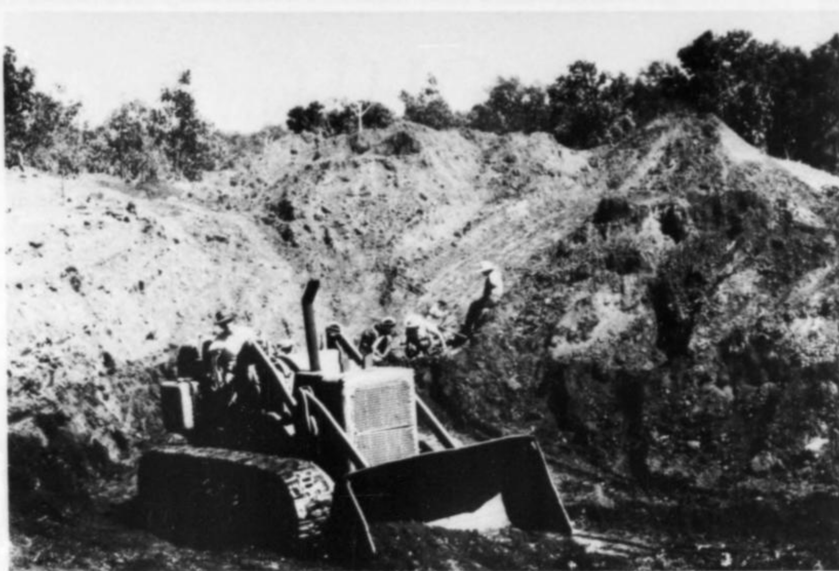
Figure 2. Excavations being made at Brown's prospect in 1973.
