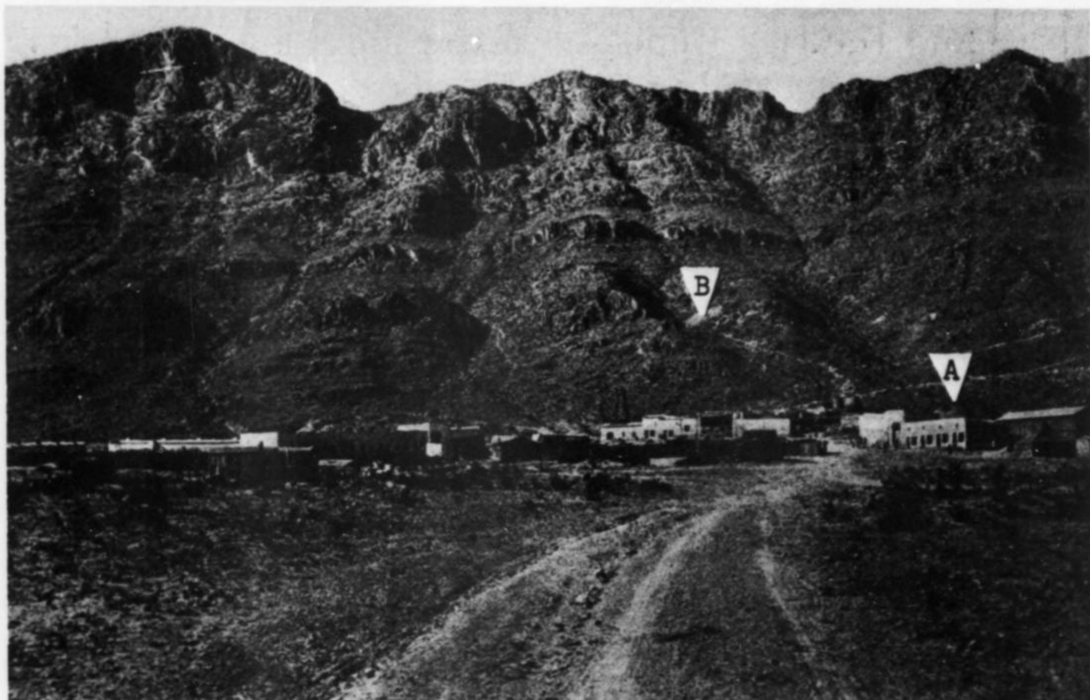
Figure 3. The Los Lamentos Range, with the locations of the Marjorie tunnel (A) and Berrenda workings (B) indicated. (From Rickard, 1924.)
