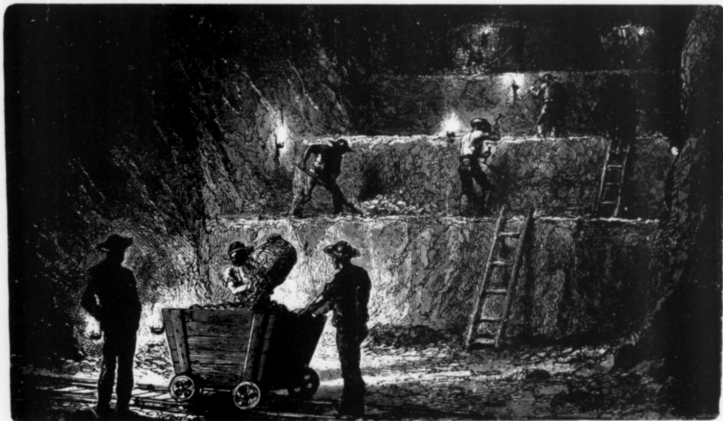
Underground benching at Stahlberg, Rhennish Prussia, in the 1860's.
