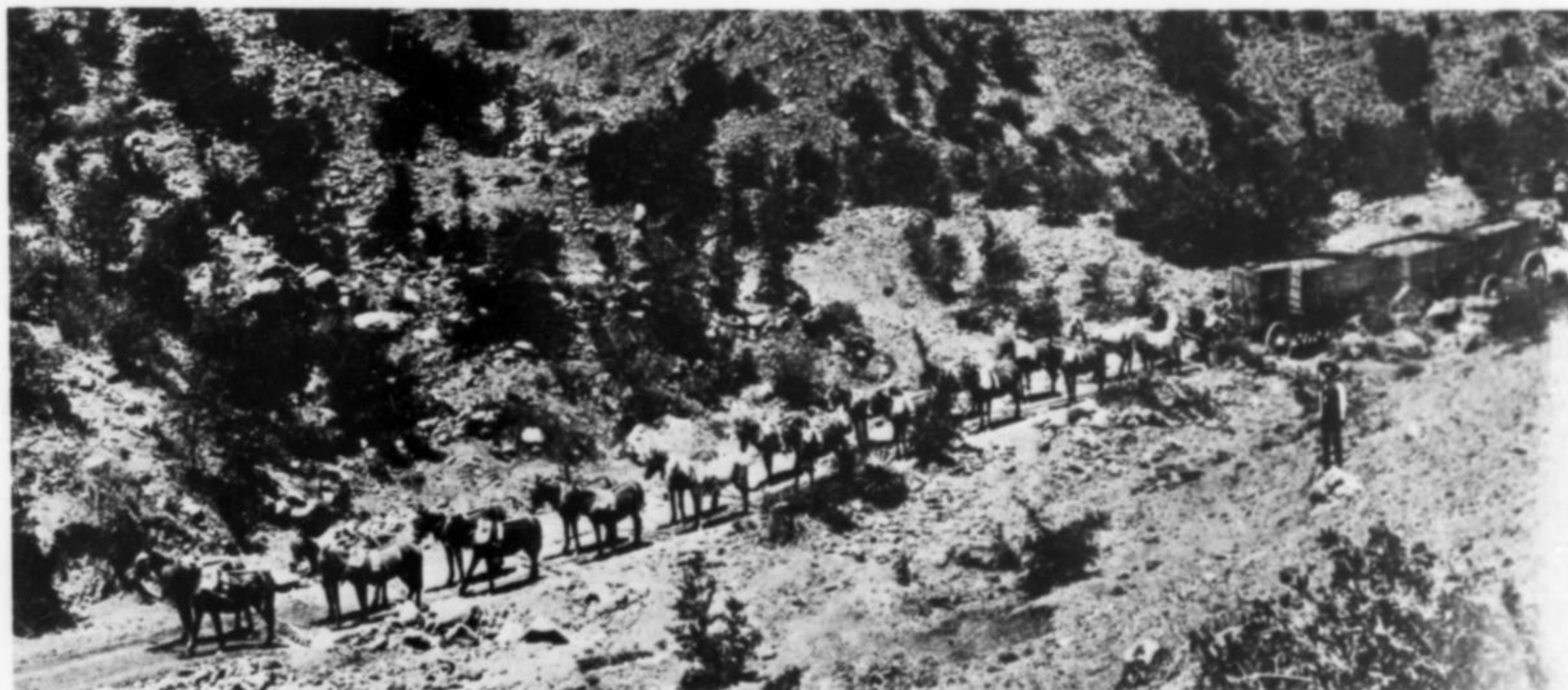
Figure 11. Ore teams of Jimmy Carr, returning to Bisbee with a load of coke. Early 1880's.
