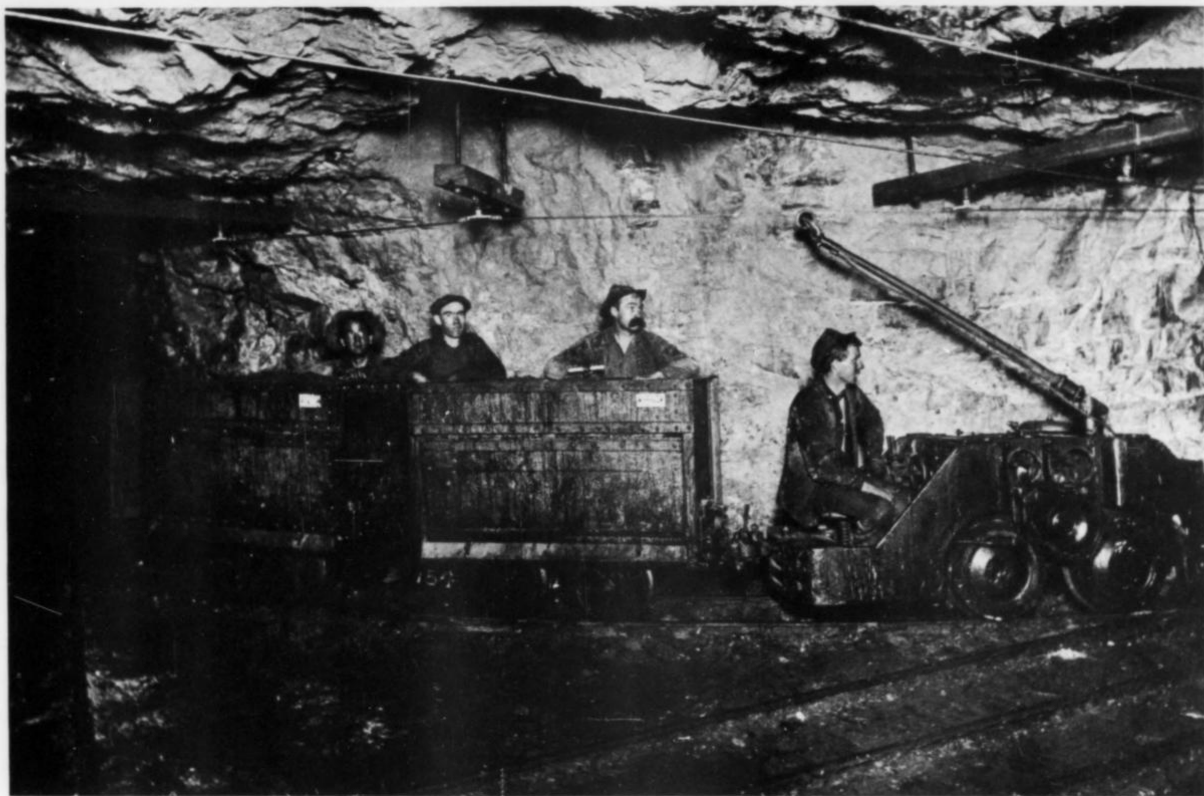
Figure 20. This electric trolley was introduced at the Holbrook mine in 1909; it is now on display in front of the Bisbee Mining and Historical Museum.
