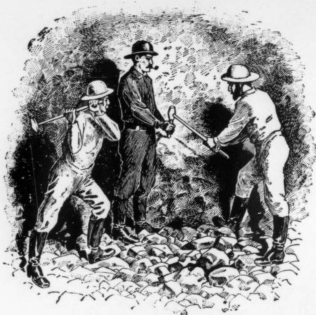
Figure 16. Three men double-jacking. The center man holds and turns the drill steel while the other two strike it with 8-pound hammers.
