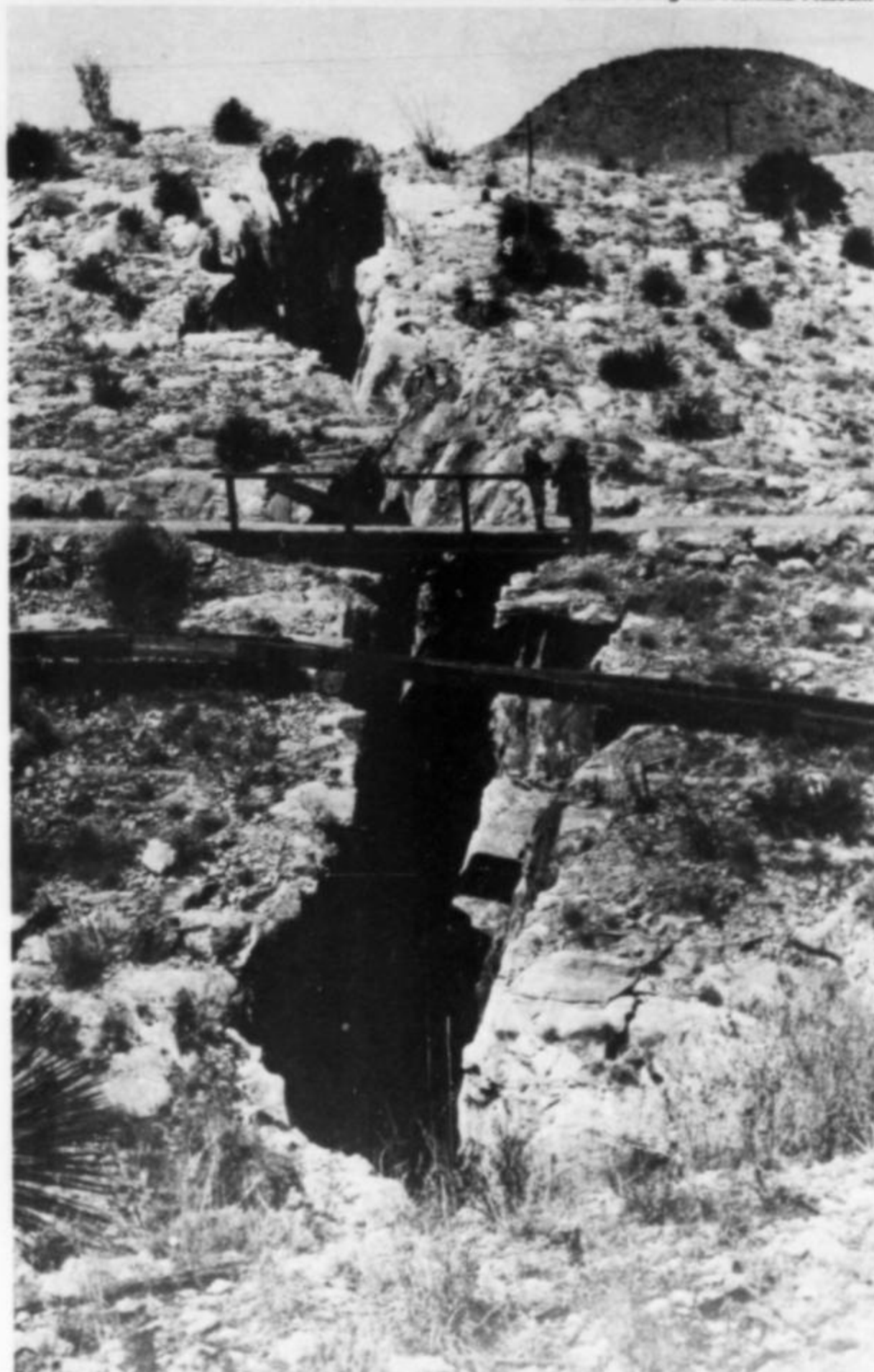
Figure 10. Surface fissures formed by subsidence due to the oxidation and later mining of copper deposits below, in the Copper Queen mine.
