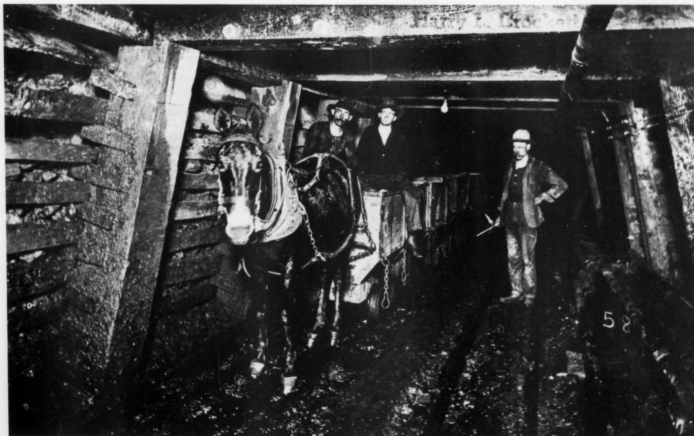
Figure 17. Mules such as this one in the Czar mine, 1908, pulled ore cars at Bisbee for many years.
