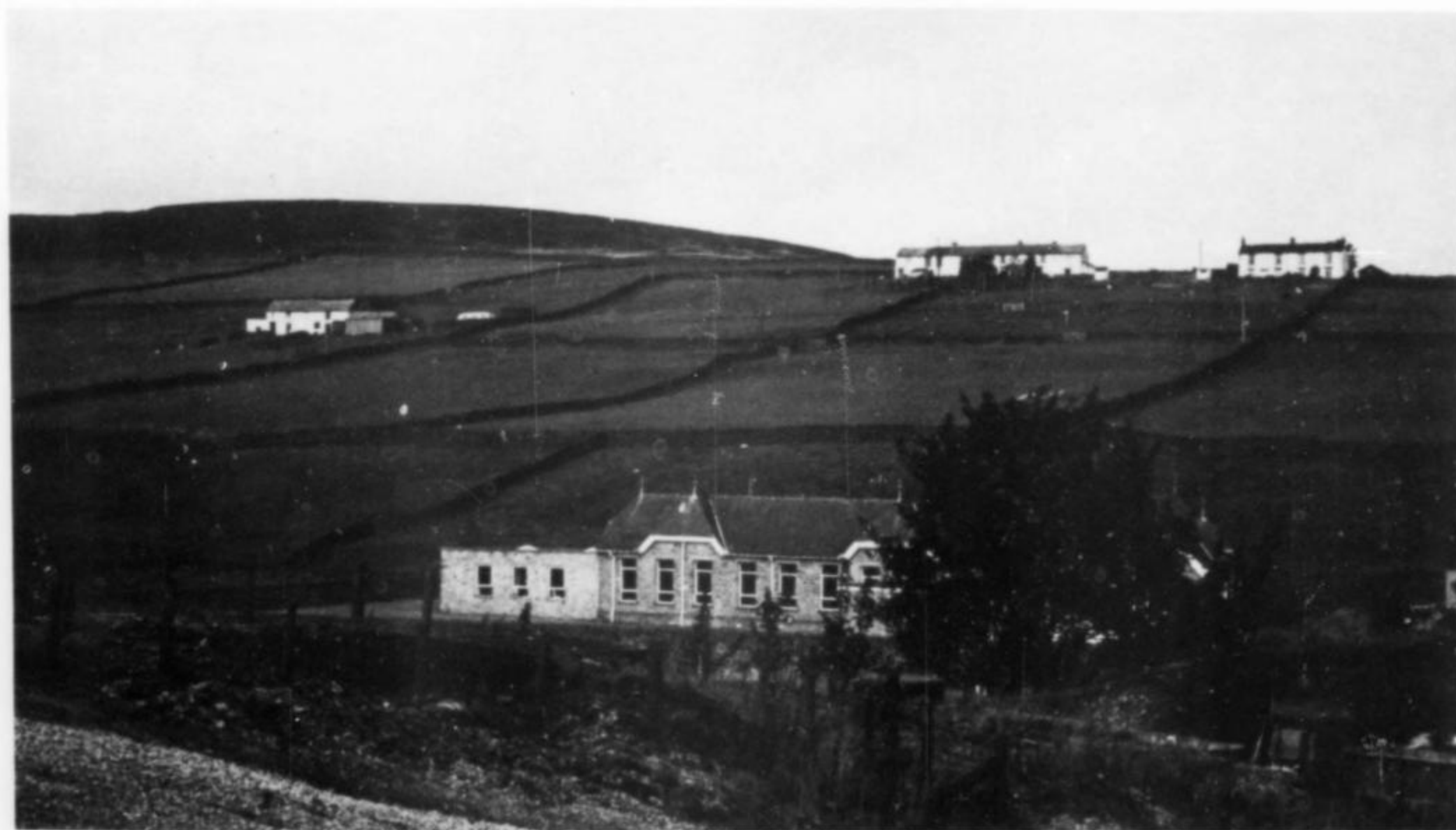
Figure 6. The Boltsburn mine in 1978, viewed from the same direction as in Figure 1. The shaft collar, covered and fenced, is visible in the foreground. The building is the Rookhope village school.
