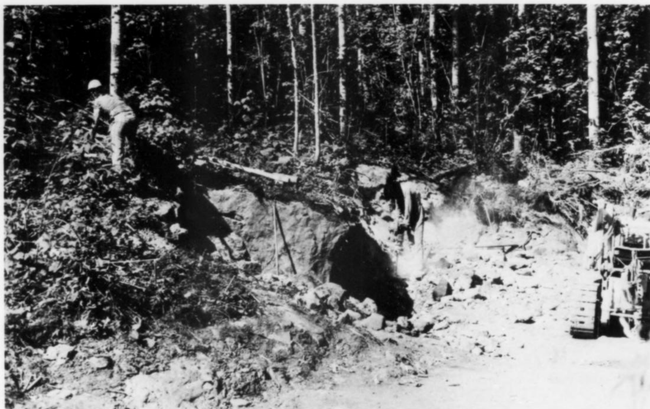
Figure 8. Clearing underbrush and drilling blast holes at the Diamond Willow mine. Photo by the author.
