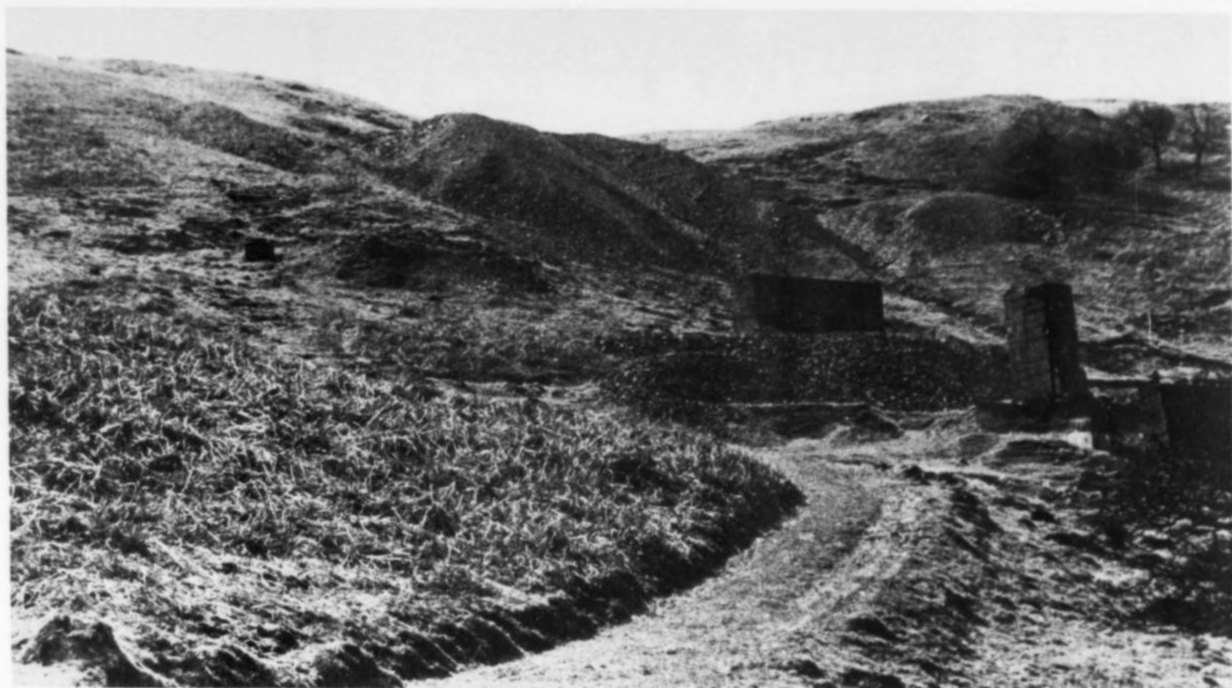
Figure 4. Bwlch-Glas mine, from the northeast. The Upper adit portal is out of sight just above the large upper dumps. (1979 photo by J. I. Wilson.)
