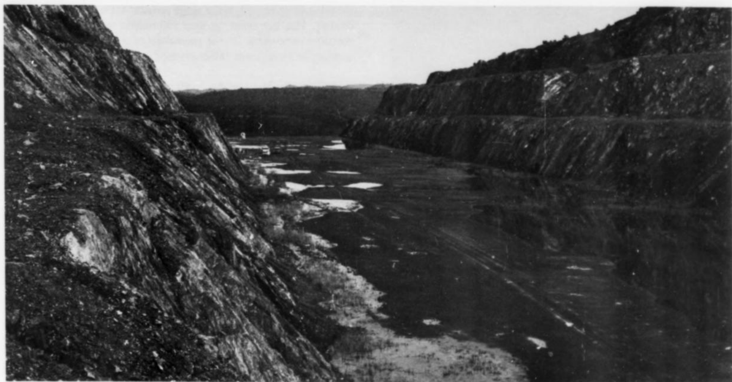
Figure 2. Spillway of New Melones Lake looking north from area 3. Benches are approximately 40 feet high.
