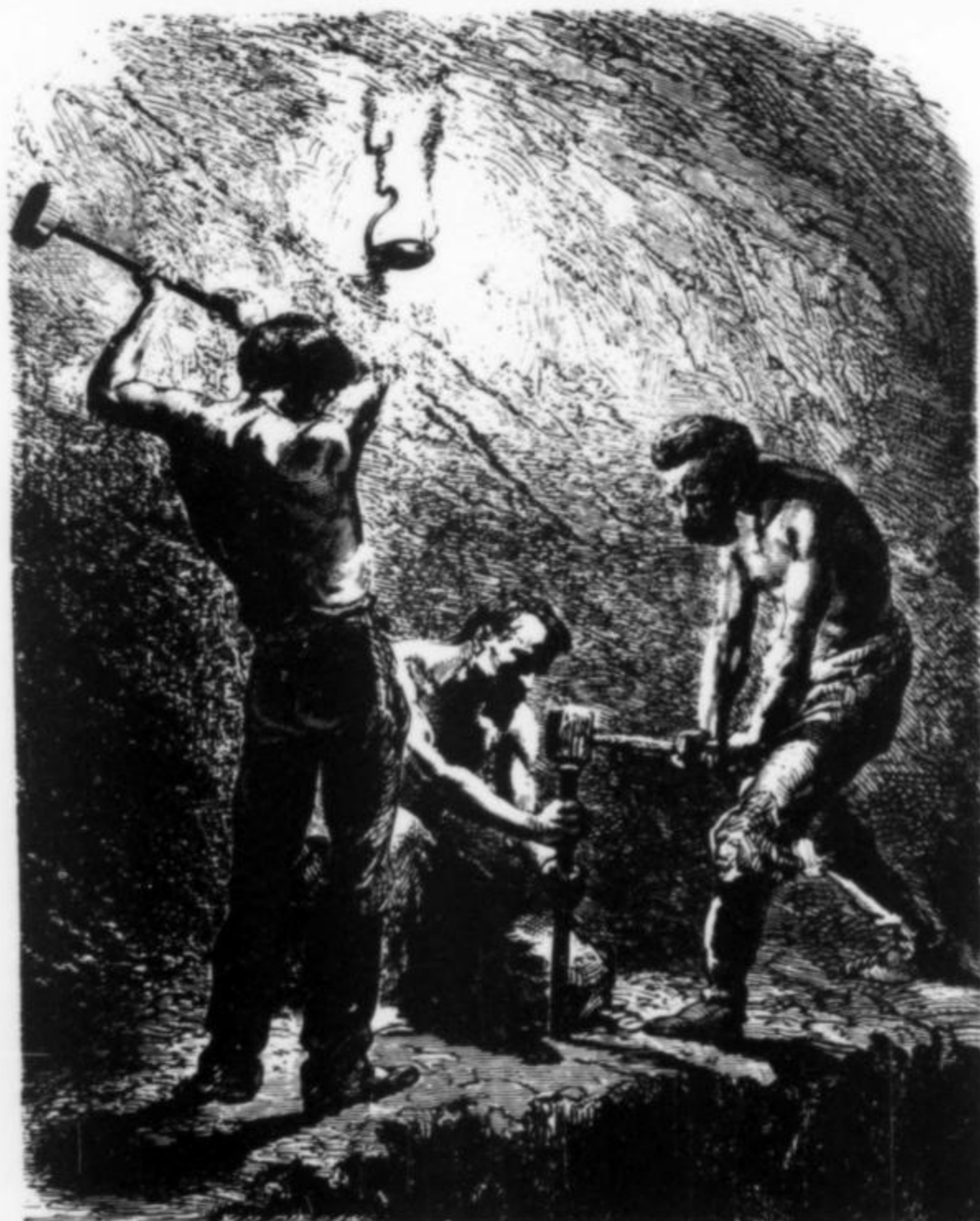
Figure 14. Double-jack drilling in the Harz Mountains of Germany, about 1860.
