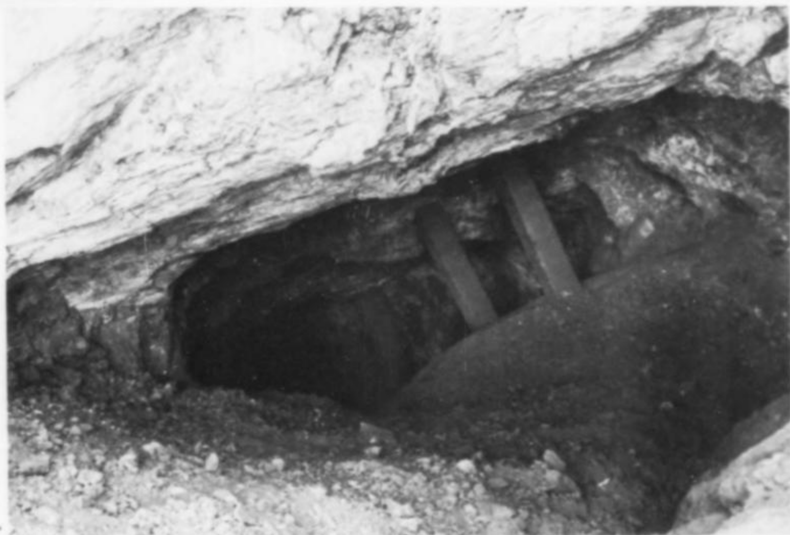
Figure 19. Looking downward into the east incline one can still see wooden stulls or timbers in place (1981 photo).
