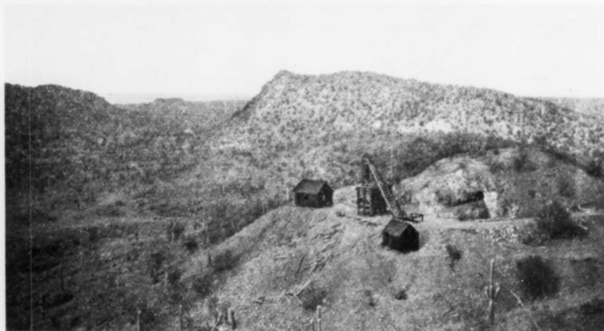
Figure 8. By 1931, as this photo taken from the west-southwest shows, the mill had been removed (Schmeltz, 1931). The headframe stands above the west incline, and two old mine buildings remain.
