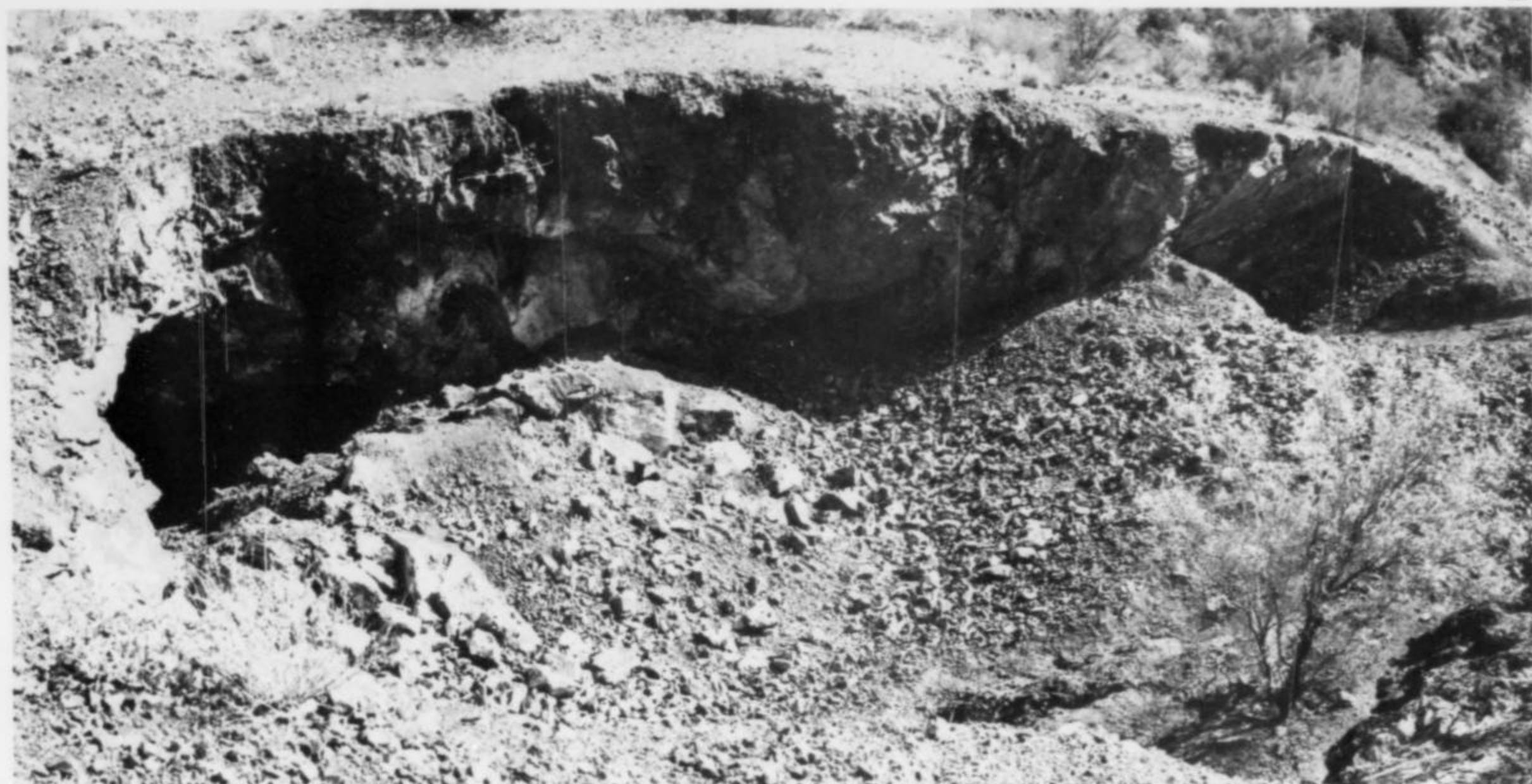
Figure 16. This photo, taken in 1981, shows the west incline entrance at far right, the smooth surface of the hanging wall clearly visible above it. Left of it is the caved and nearly blocked entrance to the glory hole stope. The photo was taken from the position marked "A" on the map of the workings, Figure 9.
