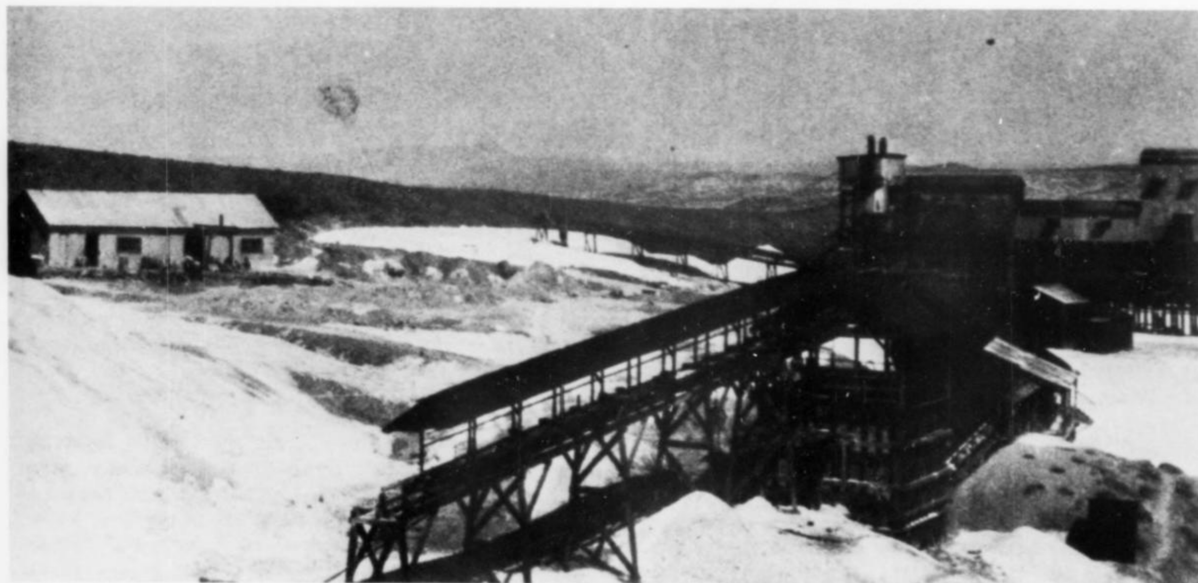
Figure 2. The mine concentrator in 1930. Photo courtesy of Edwin Sturges.
