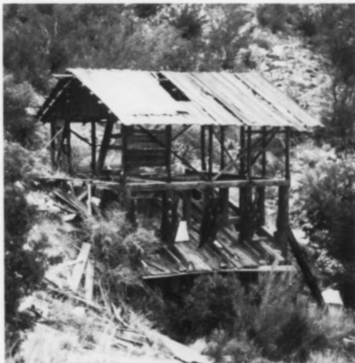
Figure 1. Old ore chutes near the Rehm dump. Miller photo.
