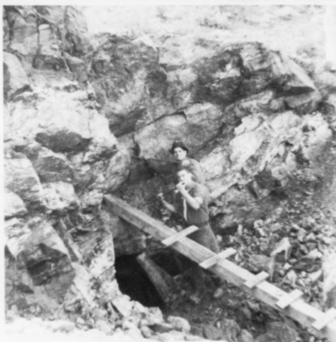
Figure 17. This photo, taken in 1957, shows the cribbing built over the entrance to the west incline. The cribbing was built to allow specimen mining in the hanging wall near where the author's 1955 wulfenite pocket was found. Later collapse of the rubble-filled cribbing resulted in the clogging of the incline below the 100-foot level. (Gene Schlepp photo.)
