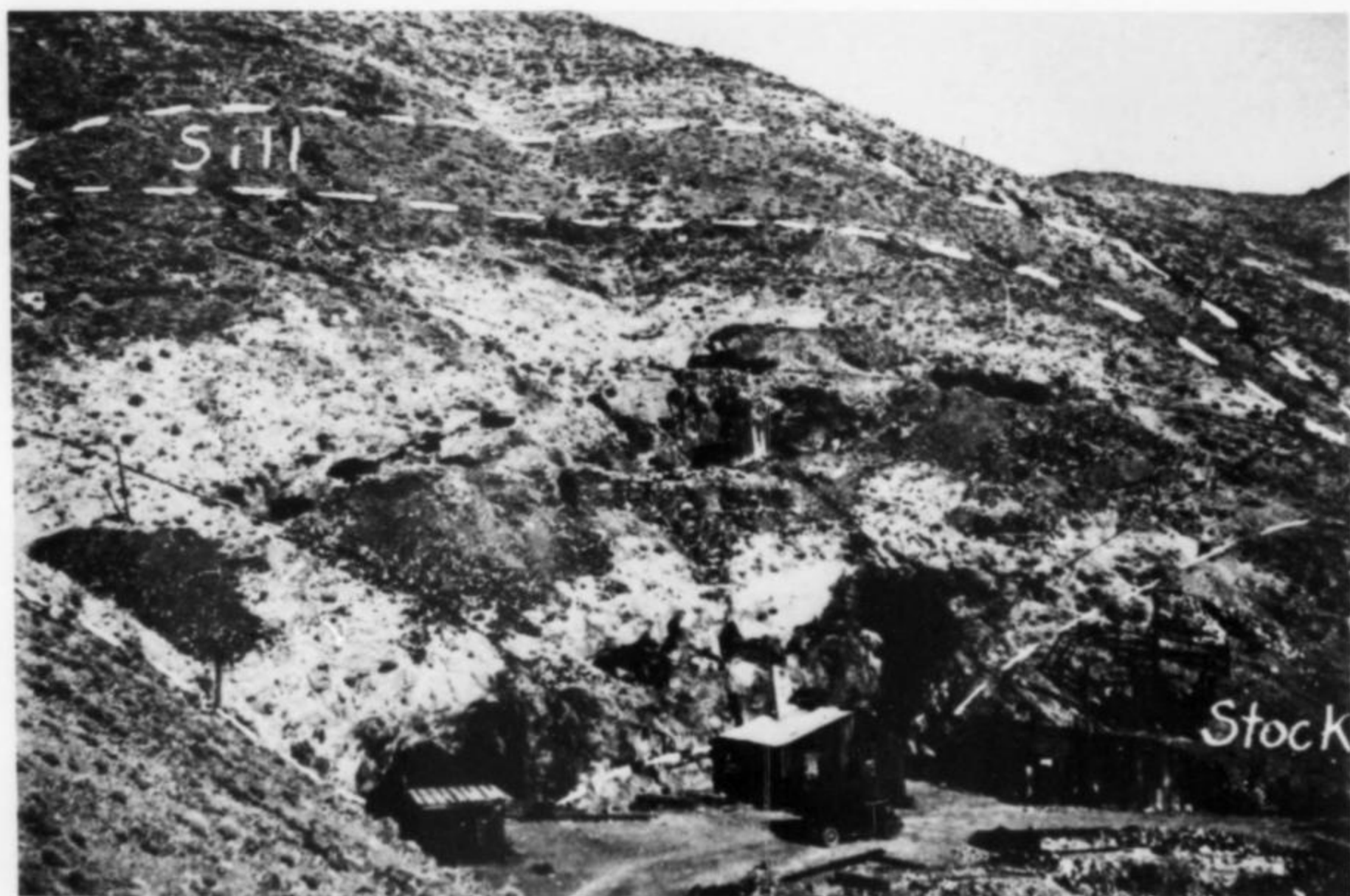
Figure 3. Defiance mine, showing the surface operation about 1936. Dr. V. C. Kelley photo.
