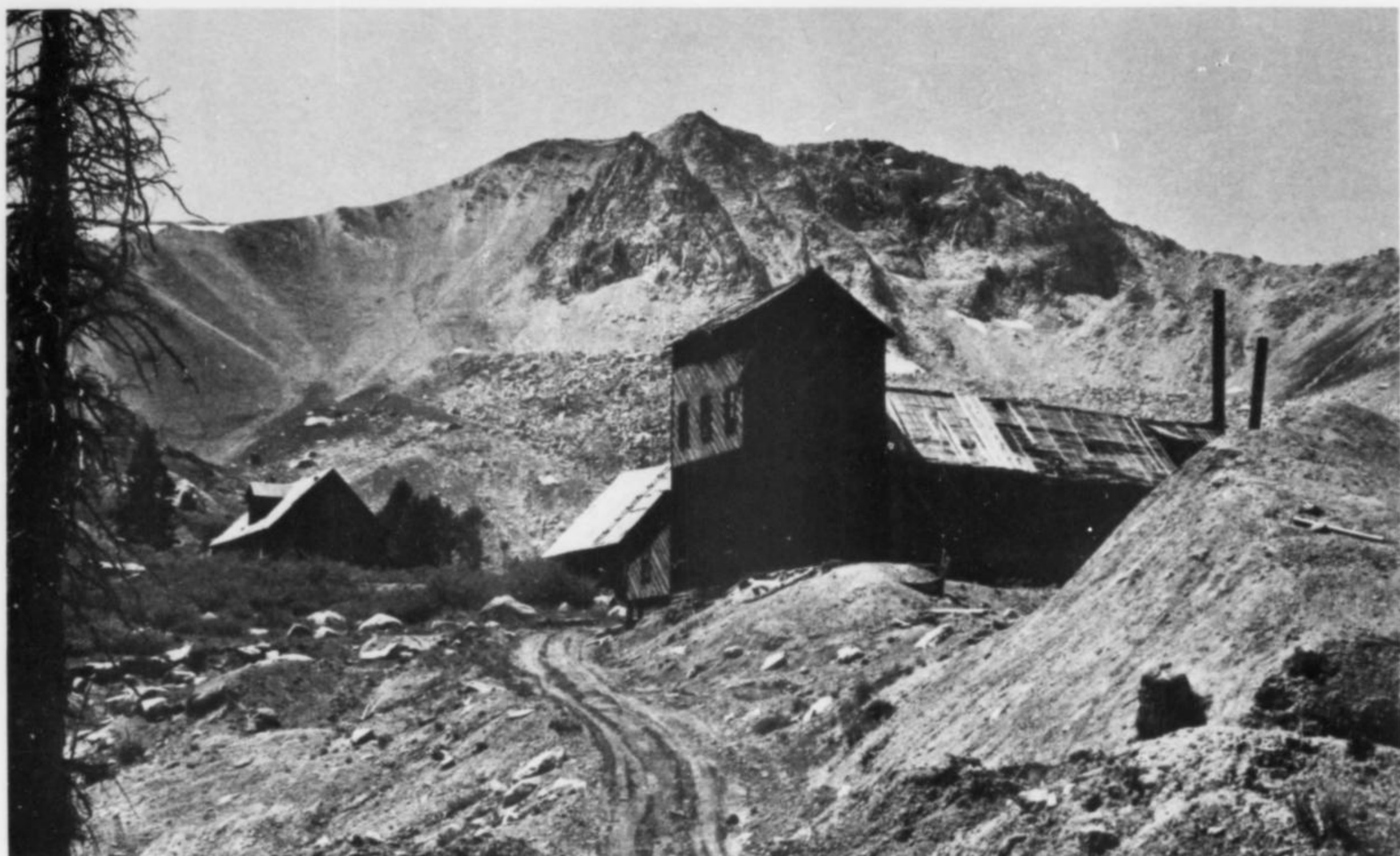
Figure 6. The Star mine, largest of the base metal mines. Italian Mountain in the background is composed of jagged rocks of the northern quartz monzonite porphyry stock in contact with sedimentary rocks of the Belden Formation (left).
