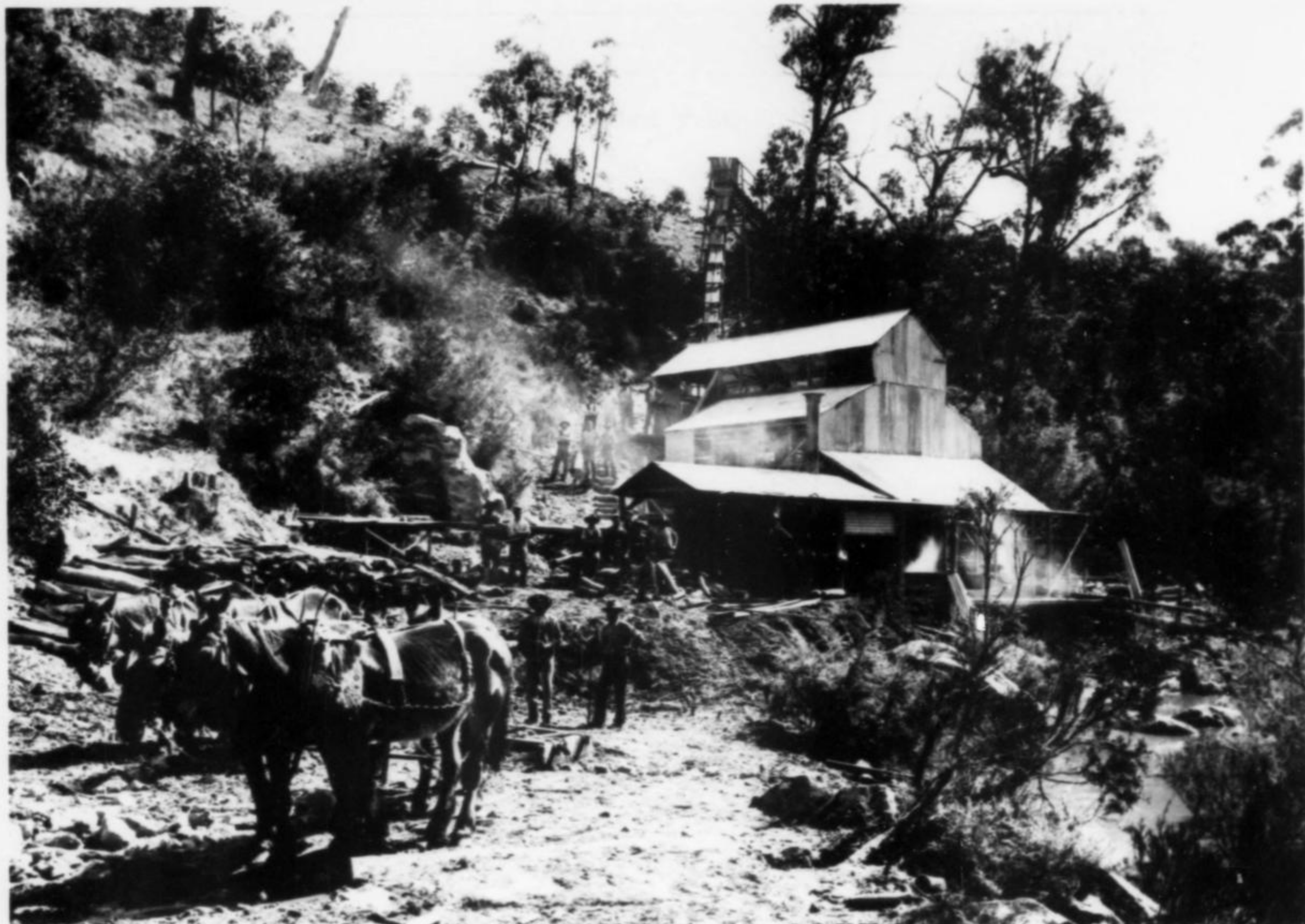
Figure 5. Sachs of Kingsgate mill, erected in 1915, showing tramway terminus and ore chute with draft horses and slide in the foreground, used to haul firewood. Photo courtesy Department of Mineral Resources, N.S.W. Government.
