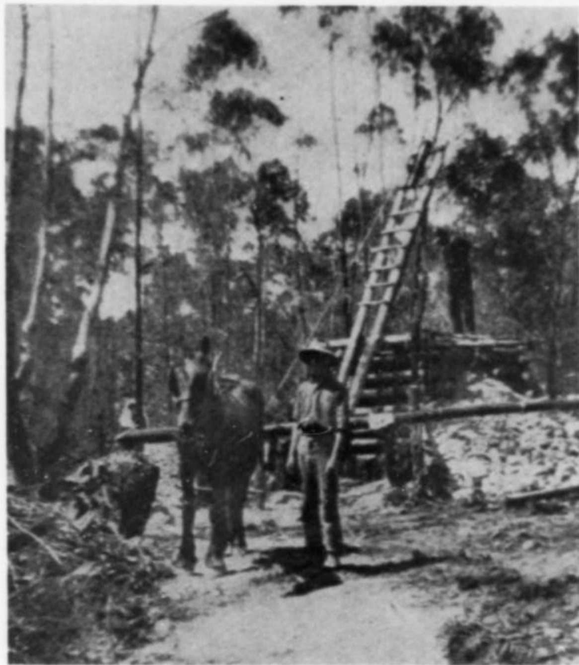
Figure 18. Vertical shaft for working No. 25 North pipe, Yates property, Kingsgate, showing improvised headframe, horse used to raise ore, and miners. From E. C. Andrews (1916).
