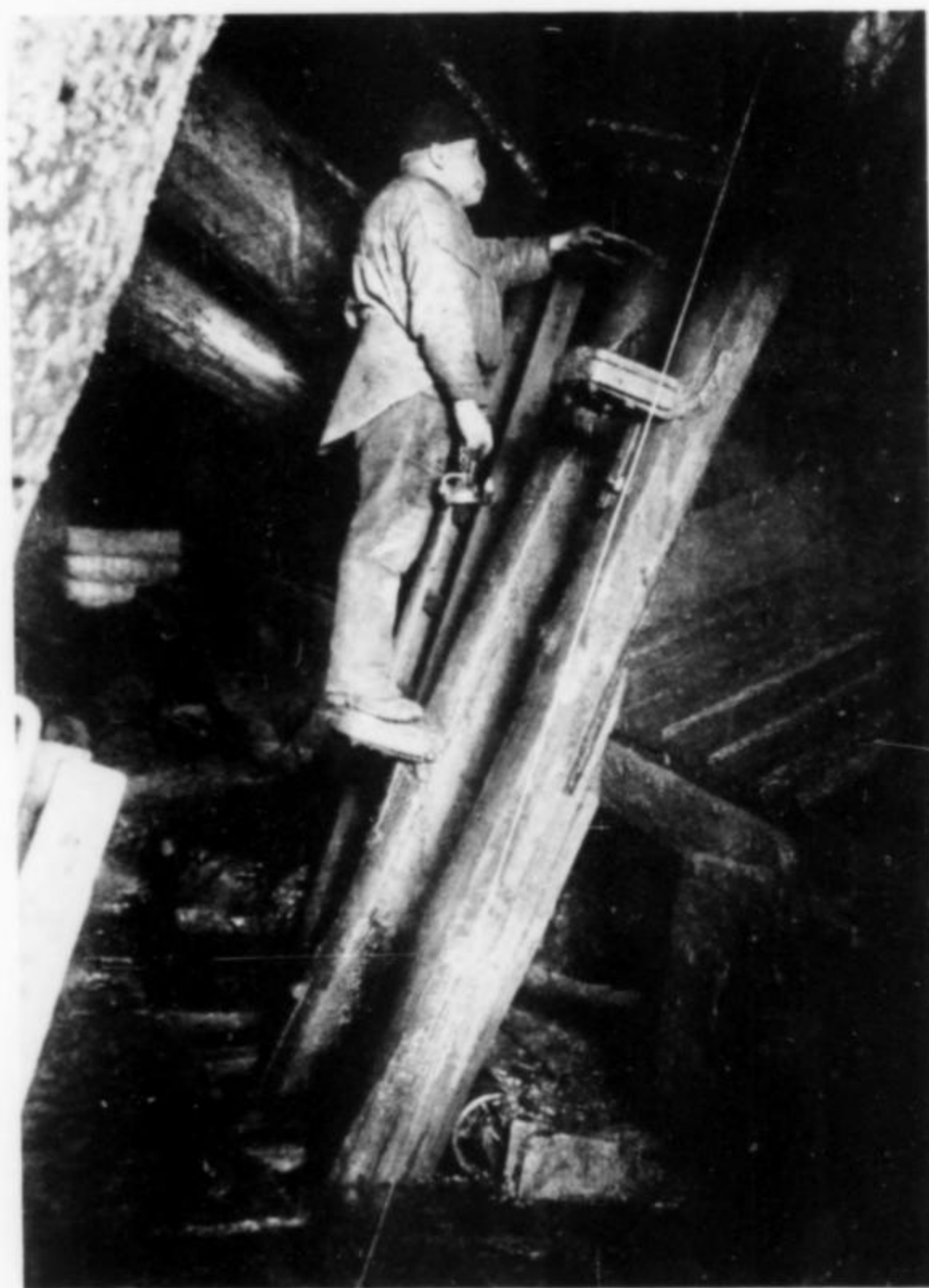
Figure 9. Miner riding the Fahrkunst in a mine at St. Andreasberg. Each pole has an up and down movement of three meters, in opposing synchronization. The miner steps back and forth between the poles, catching each one at the bottom of its swing, and rides up the shaft.
