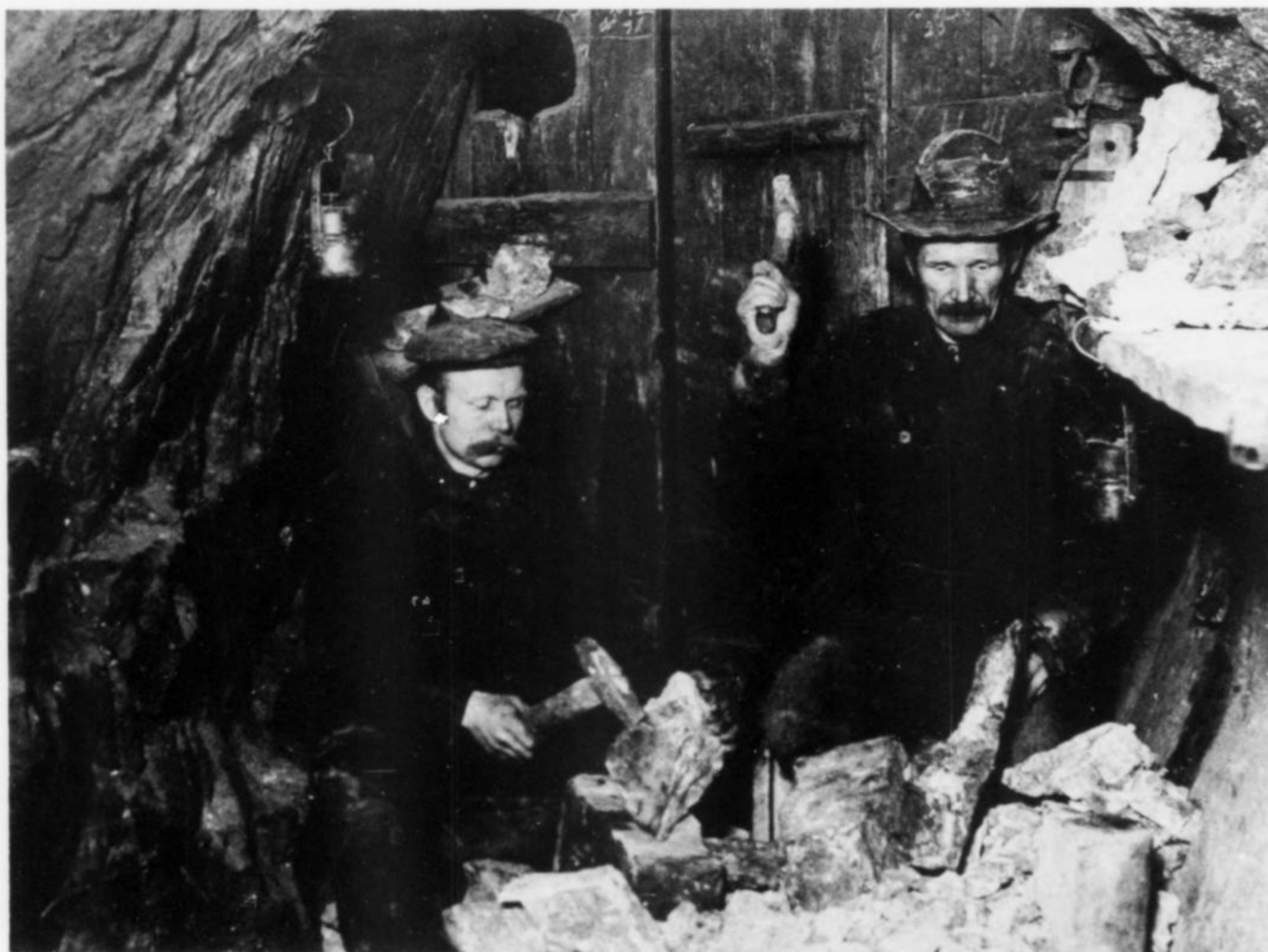
Figure 5. Miners cobbing out native silver in the Samuels mine, ca. 1900 (courtesy Kongsberg mining museum).
