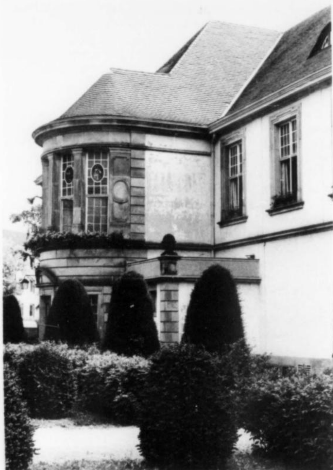
Figure 2. Portion of the show building.
