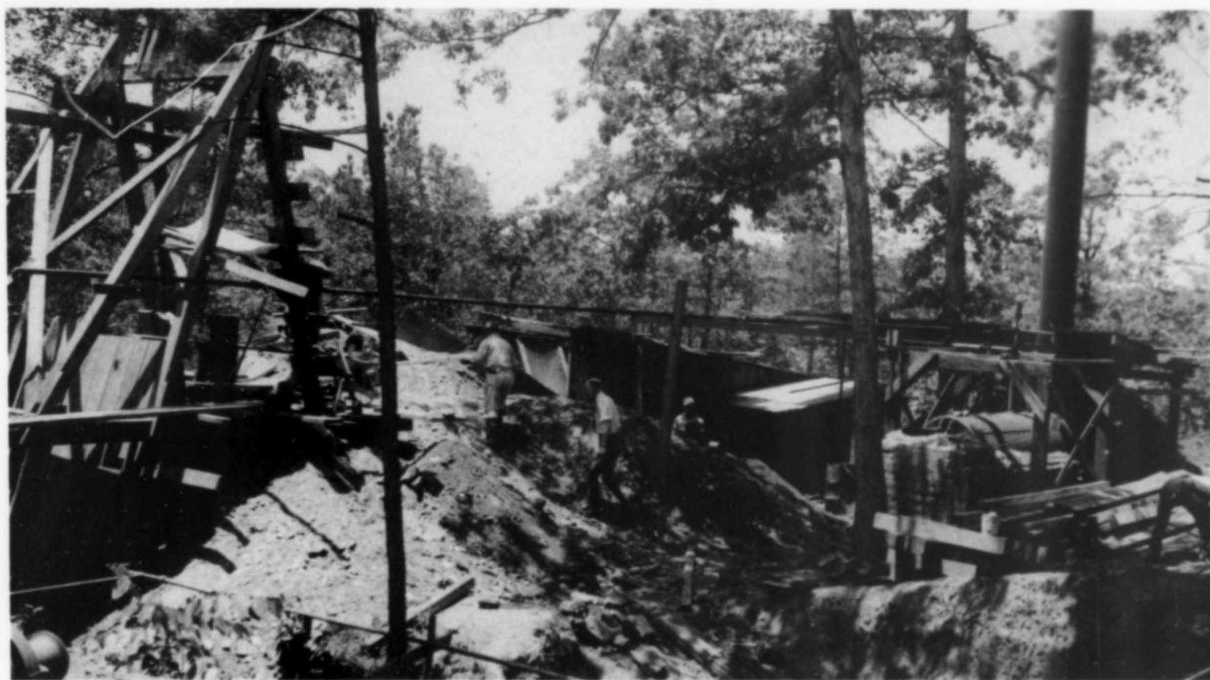
Figure 2. Depression-era attempt to reactivate the 301 mine, 2 km west of Holly Springs, Cherokee County, Georgia. This unsuccessful effort was typical of many such operations in response to $35/ounce gold and the high unemployment of the early 1930s. Note the archaic steam boiler being used for mine power. Photo by R. W. Smith, June, 1934.
