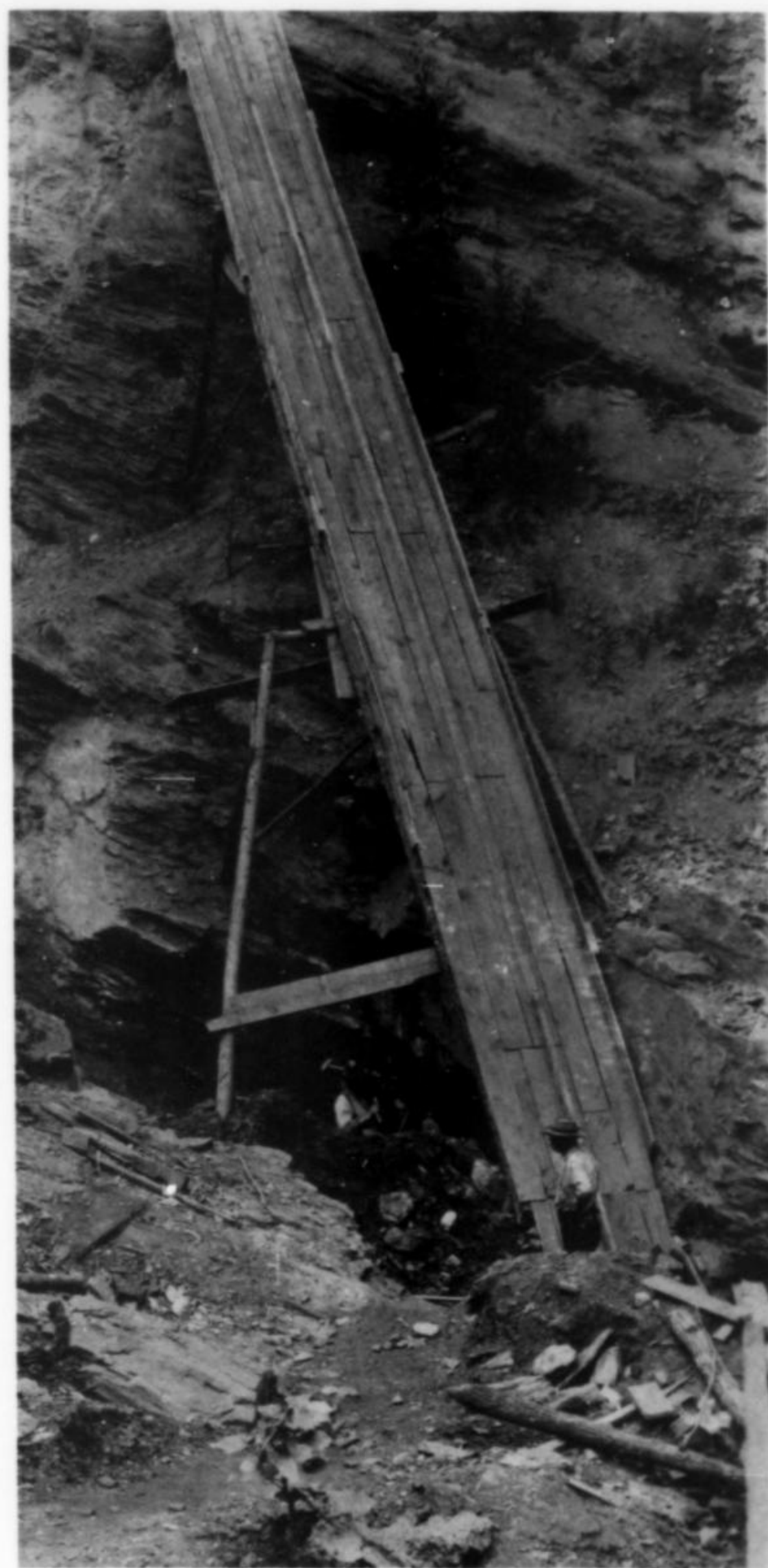
Figure 5. Inclined skipway to a shaft on the main ore shoot in the Findley mine open cut, Lumpkin County, Georgia. Photo by S. W. McCallie, August, 1913.
