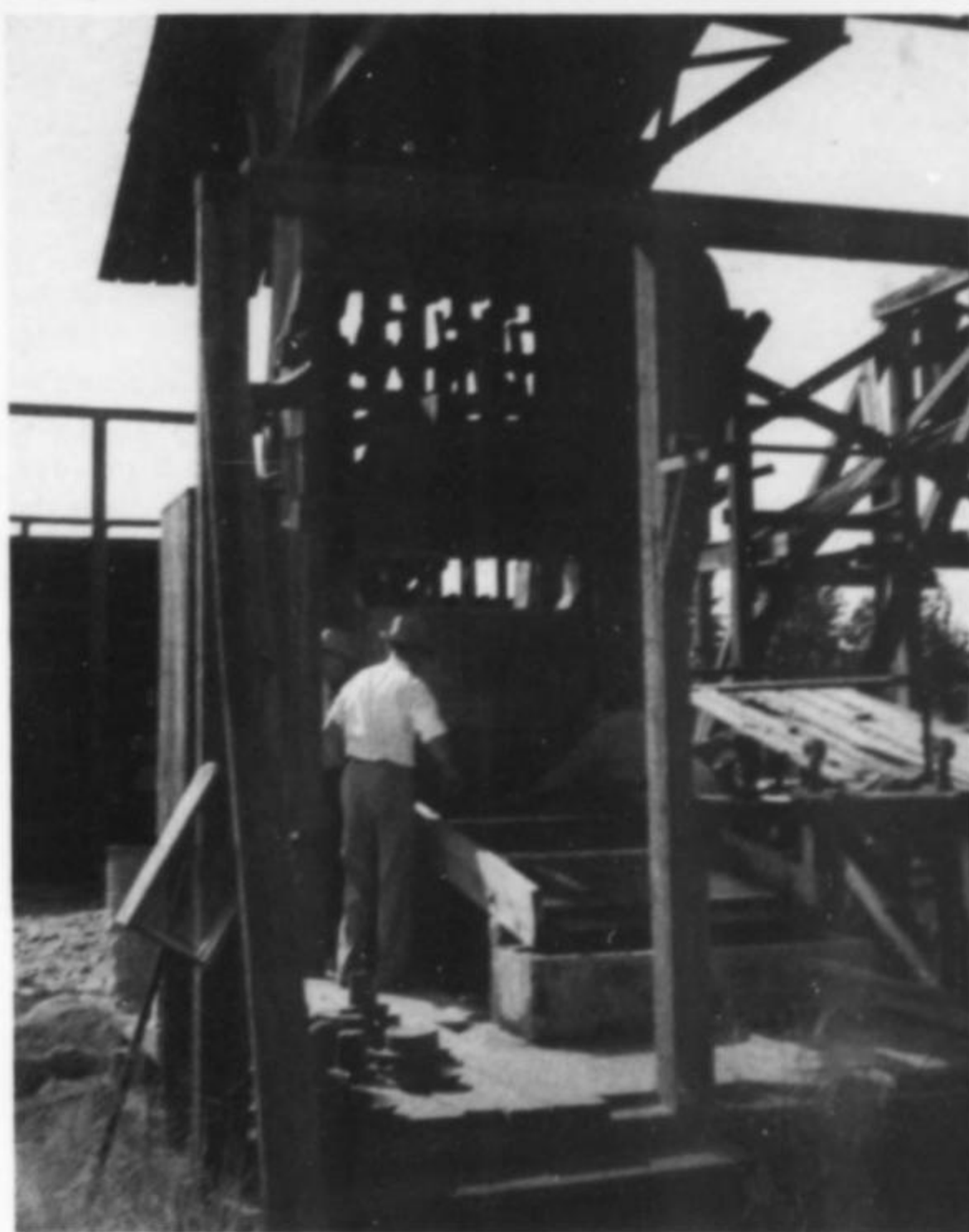
Figure 3. The last successfully operated production stamp mill in Georgia. This mill was operated at the Fluker (Columbia) mine in McDuffie County until the federal government forced its closure during World War II. Photo by A. C. Munyan, September 11, 1939.
