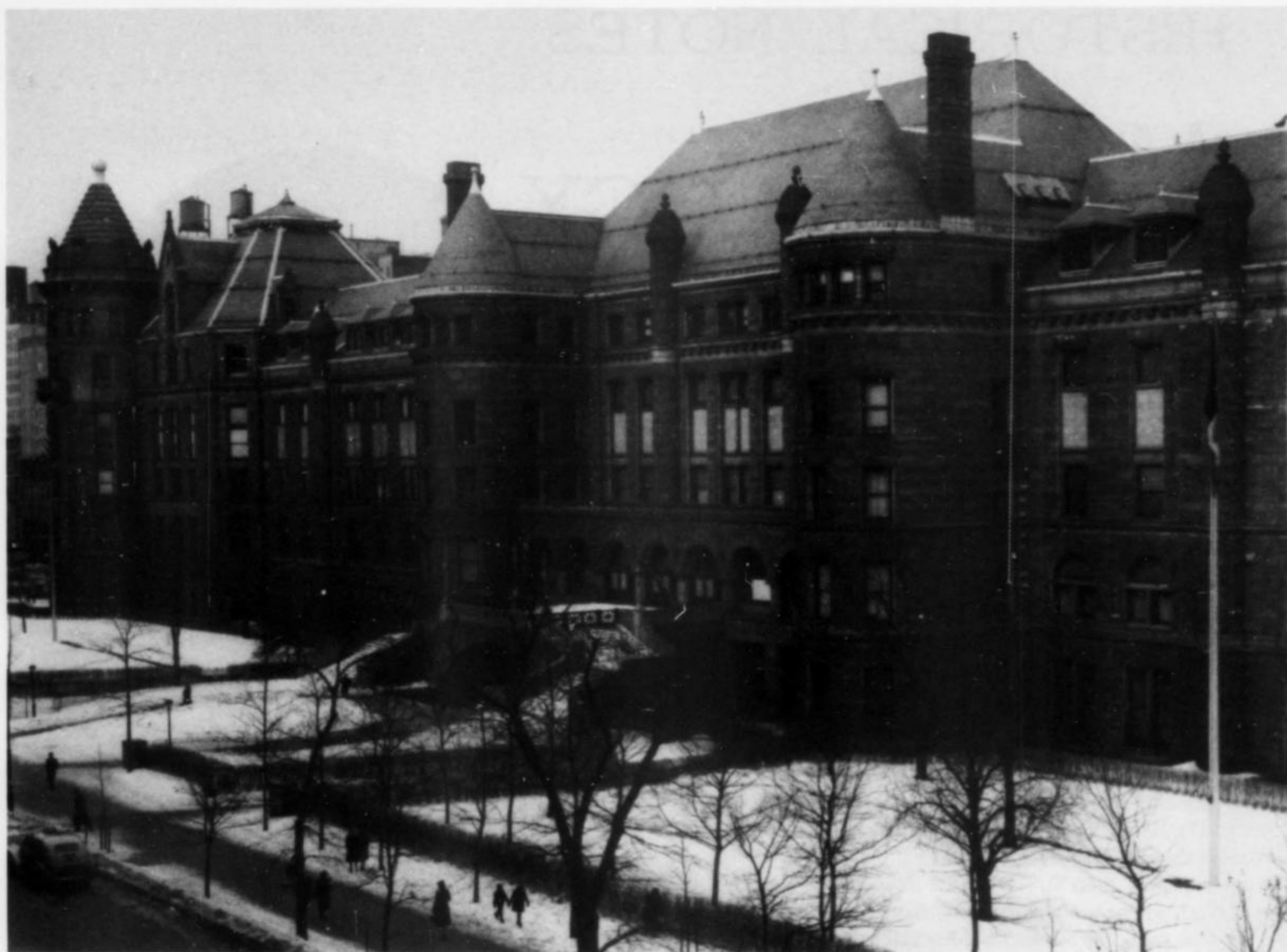
Figure 2. South facade of the American Museum of Natural History in New York, early 1940's. Photo by Dwight Bentle.
