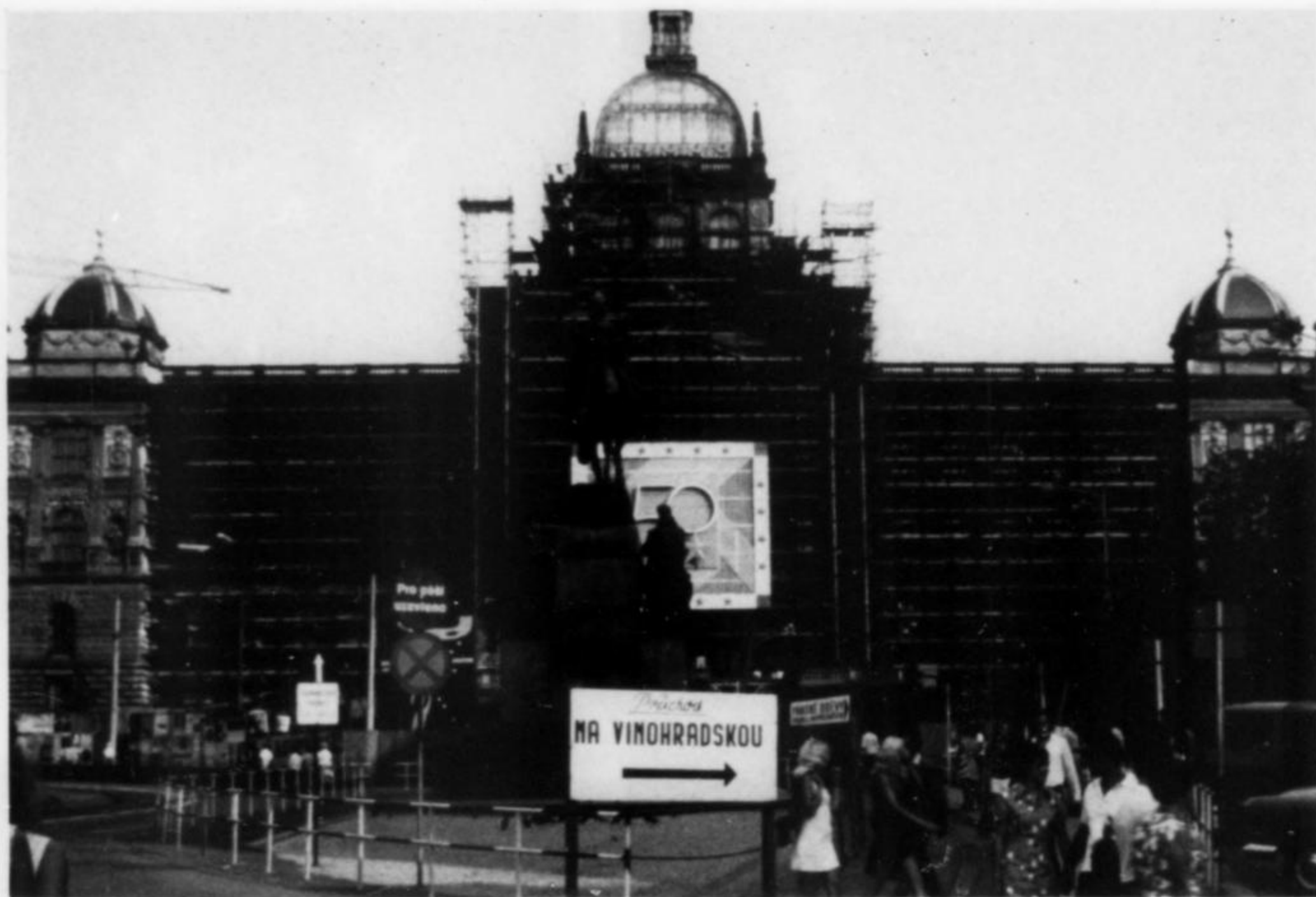
NARODNI MUSEUM Facade under reconstruction
