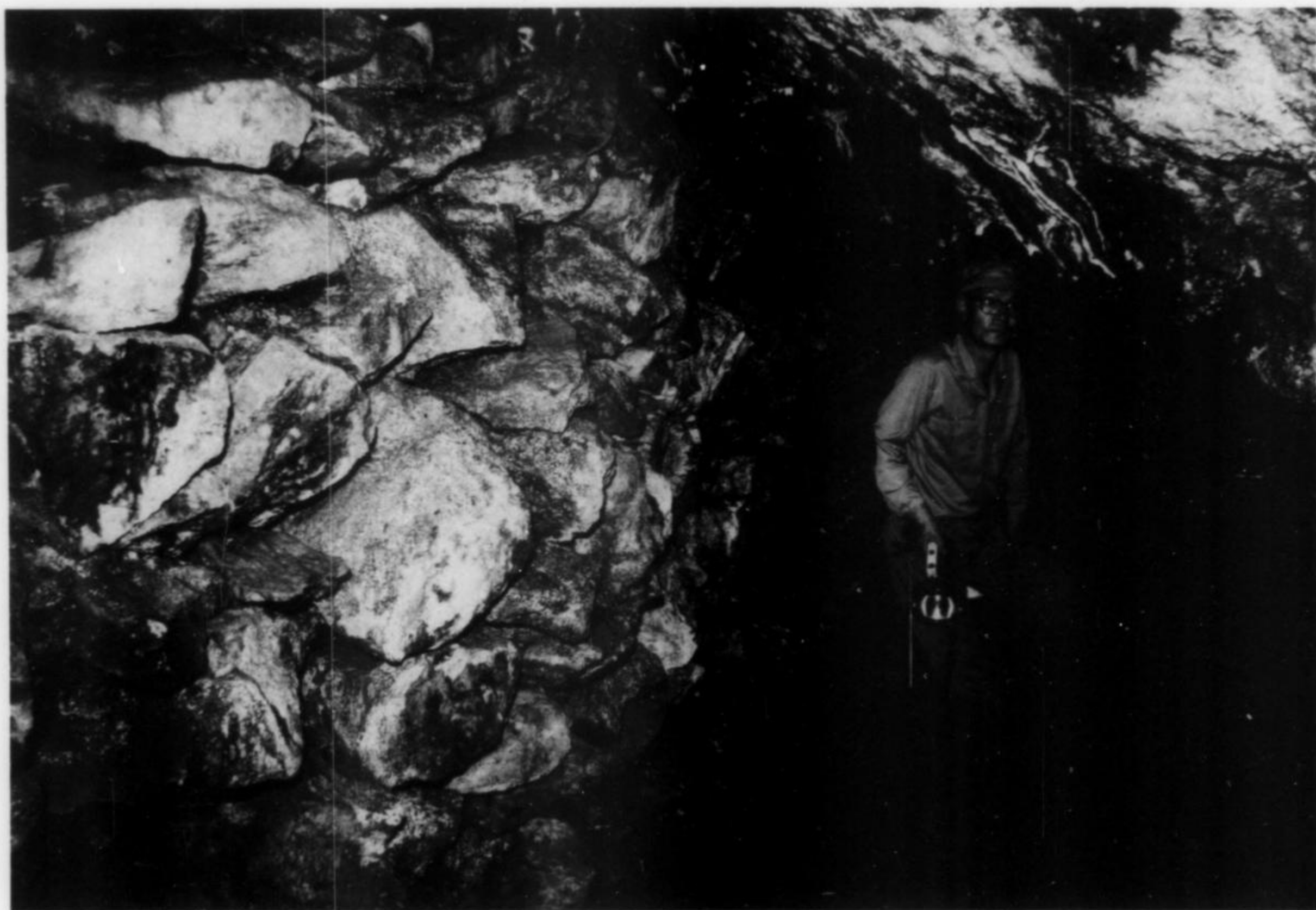
Figure 16. Century-old neatly stacked rock wall still supporting mine ceiling. Bancroft photo.
