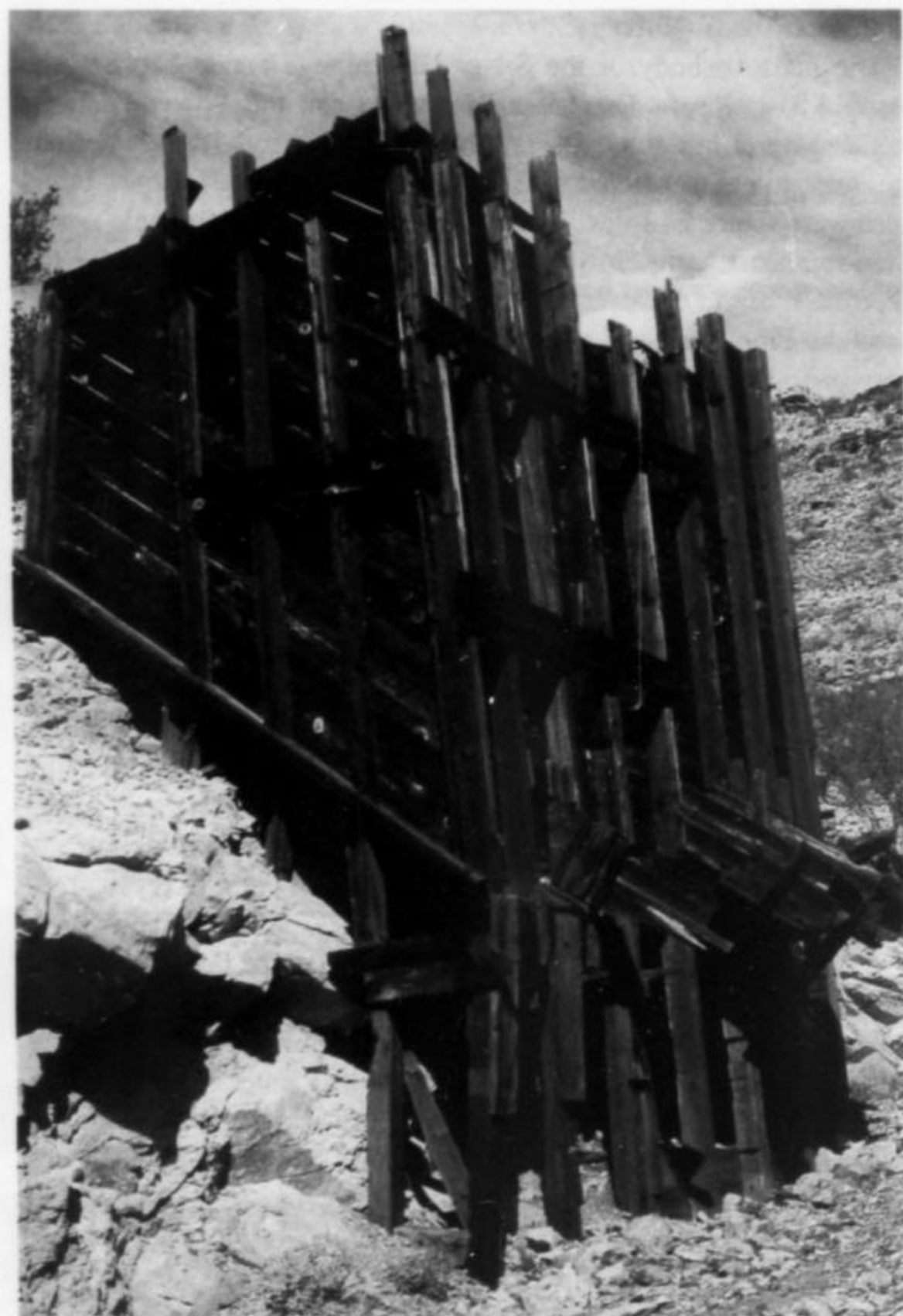
Figure 2. Ore bins at the Silver Hill mine.
