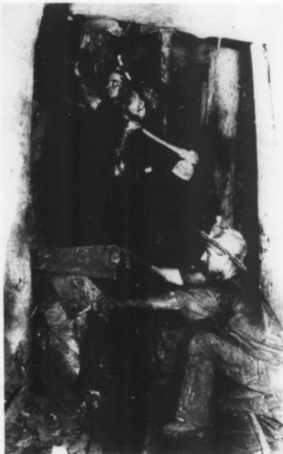
Figure 9. Underground at the Moonta mines, circa 1910. Timbermen replacing timber in a drive. (Mortlock Library B24094)
