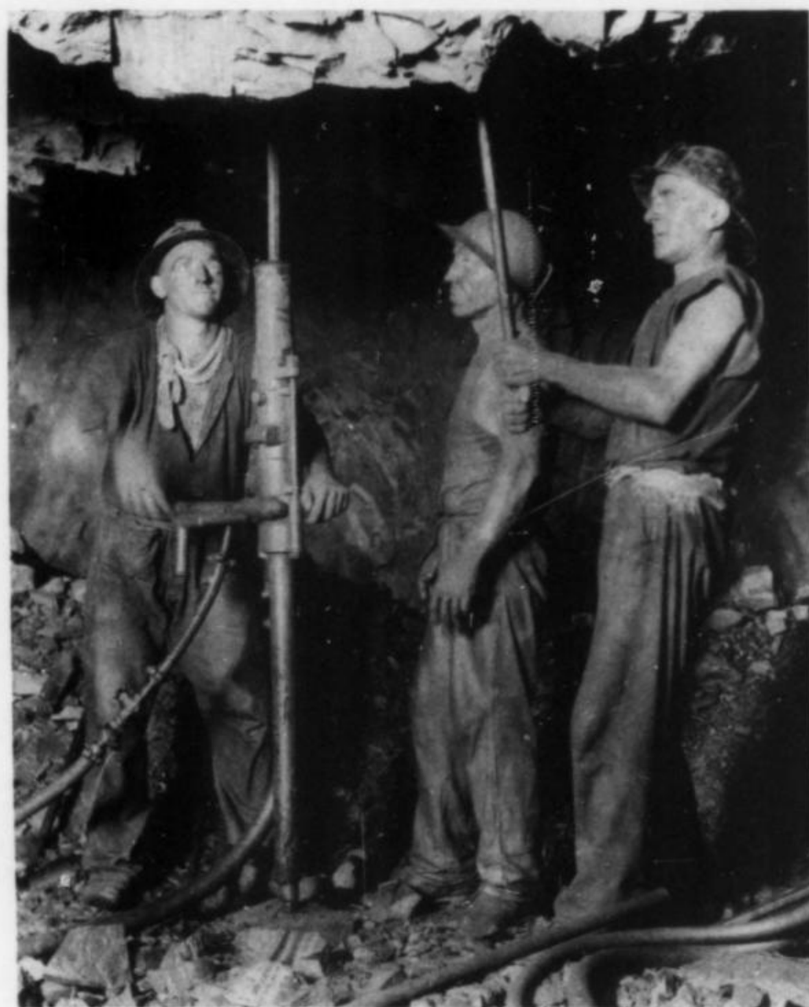
Figure 10. Shrinkage stoping in the Black Rock area, Mount Isa, in 1932. Photo courtesy Mount Isa Mines Ltd.
