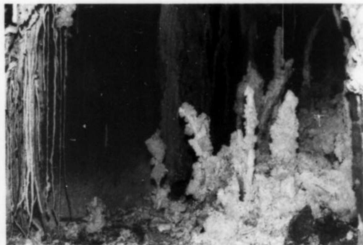
Figure 19. Post-mining growths of sulfate minerals on 4 level, Mount Isa mine. The filaments at left are about 1.5 meters long. Photo by the author.
